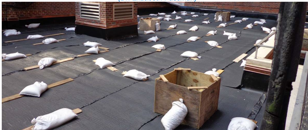
Figure 10. Drainage layer held in place with sand bags (Dr. Elizabeth Fassman)
