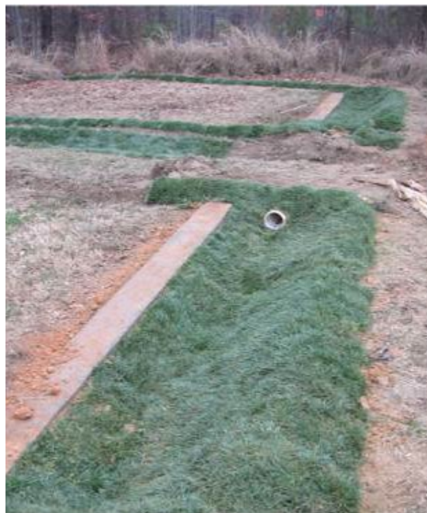
Figure 11: LS and Blind Swale Post-Construction
