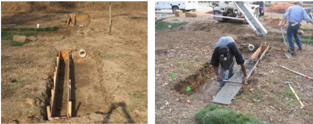
Figure 10: Forming the Level Lip (NCSU-BAE)
