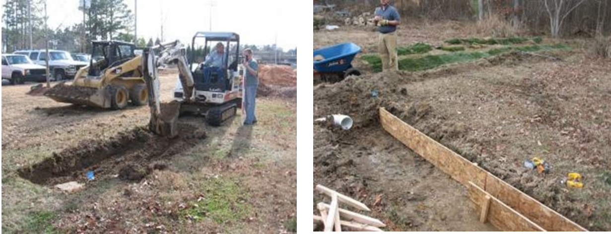
Figure 9: Excavating the Blind Swale (NCSU-BAE)
