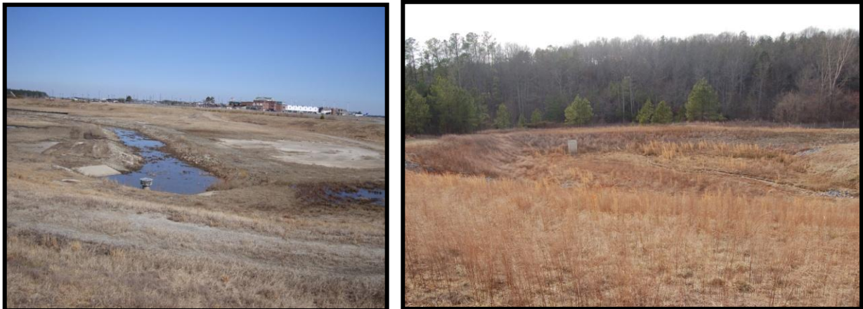
Extended dry detention basin at airports in Wilmington, NC (left) and Concord, NC (right).
