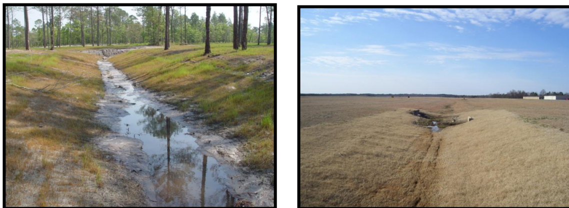
Grassed swales at a Brunswick County development (left) and the Harnett County Airport (right).
