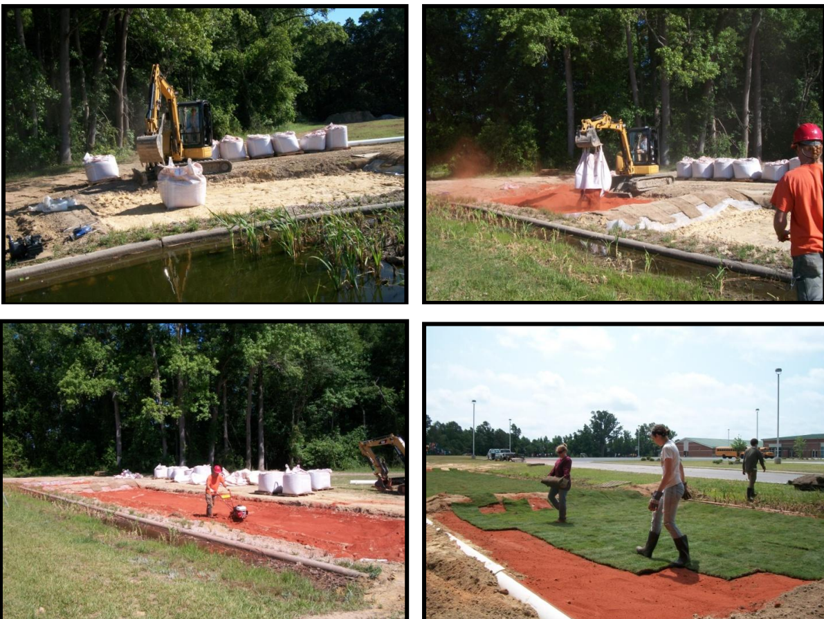
Installation of soil amendments in a vegetative filter strip
