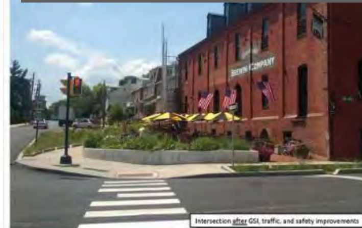
Intersection after GSI, traffic, and safety improvements
