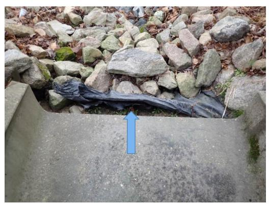
Fabric not folded and tucked properly beneath the outlet flared end section (FES)
