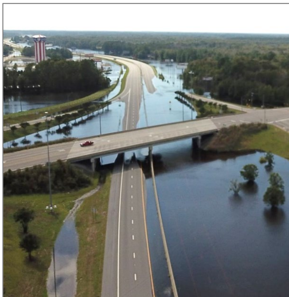
Flooding of I-95 in Robeson County
