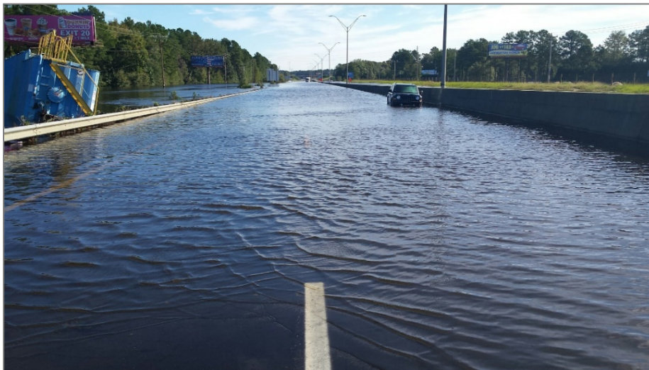
I-95 Flooding at MM 18 in Robeson County after Hurricane Matthew
