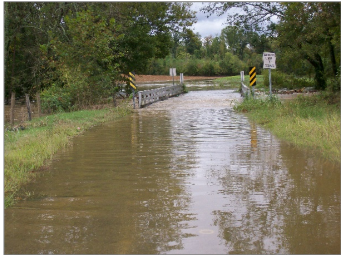
Roadway flooding after tropical storm Nicole
