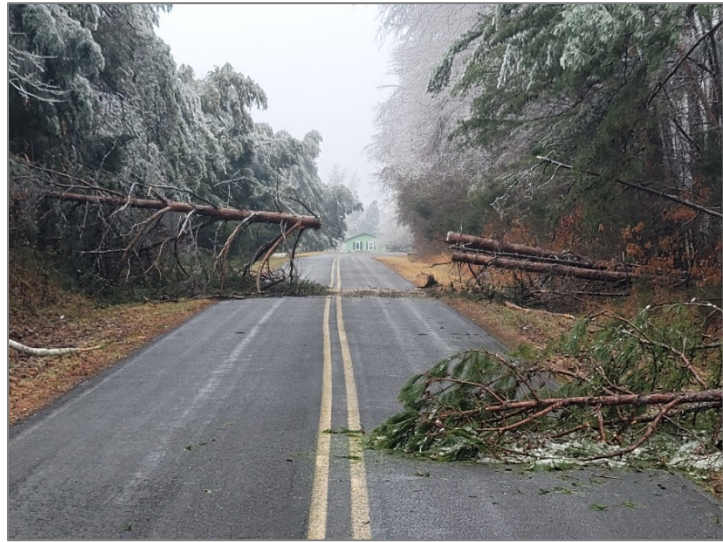
Ice damage in Granville County
