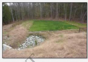
VFS is placed into one of four categories: protected riparian buffer, wooded stormwater setback/buffer, herbaceous stormwater setback/buffer, or engineered filter strip. The VFS is usually 30 feet in width except when the LS-VFS is used to meet stormwater rule requirements in SA waters, in which case the VFS must be a minimum of 50 feet in width.
