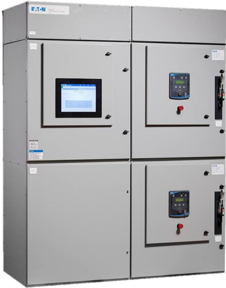
Medium Voltage Control
