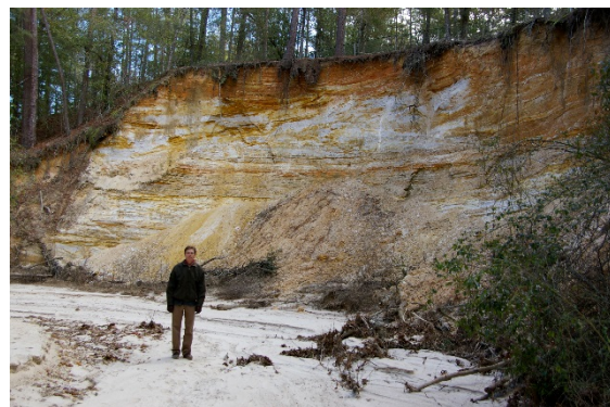
Exhibit 23. Stormwater has eroded a deep canyon in the banks of the Sand River.
