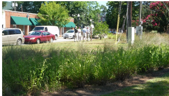
Exhibit 25. Rain gardens in street medians help manage stormwater while providing attractive landscaping.
