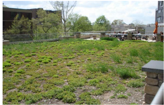
Exhibit 19. The green roof system on the Radian Complex diverts stormwater from the combined sewer system while giving residents an attractive view.
