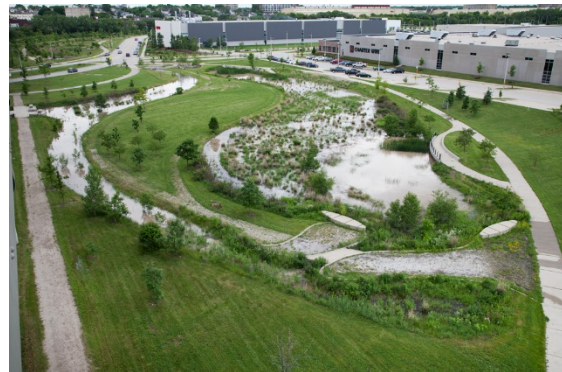
Exhibit 28. The MVIC Stormwater Park manages stormwater runoff while providing a new public space with pedestrian and bicycle trails.
