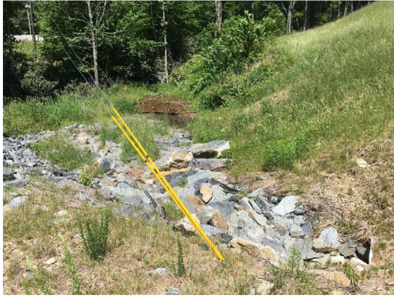
Stormwater feature on the northern portion for future enhancement, facing northeast
