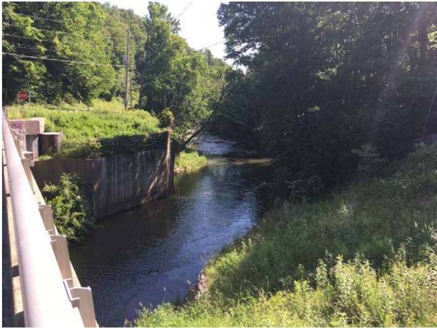
North portion from Old Blowing Rock Road, facing north
