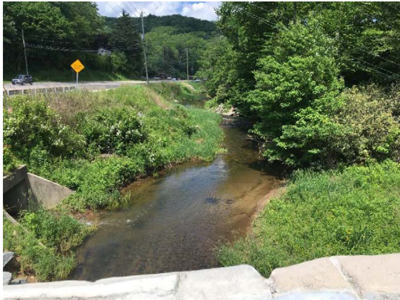
North-central portion at Chestnut Ridge Bridge, facing north
