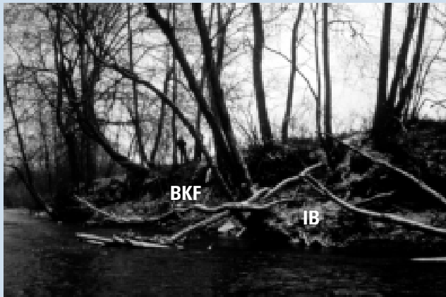
2a. Mills River Gage, Henderson County, C4 stream type. The break in slope at the lower bench is the inner berm (IB). Bankfull (BKF) is the upper scour line.
