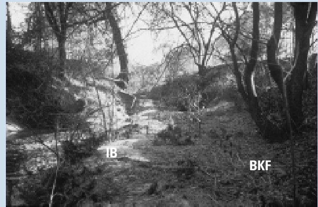
2b. Rocky Branch, Wake County, G4/F4 stream type. This stream is actively building a new floodplain. The front of the bench is the inner berm and bankfull is the back of the bench.
