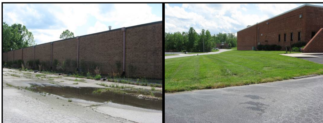
Figure 46. Photographs taken in the Nance (High Point) watershed depicting industrial land use characteristics.
