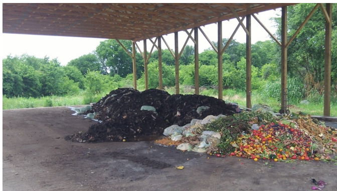
A fresh load of food residuals are dumped on the concrete pad of Gallins Family Farms' composting operations (shown above). It will be mixed with carbon material and formed into a windrow for the composting process to begin.
