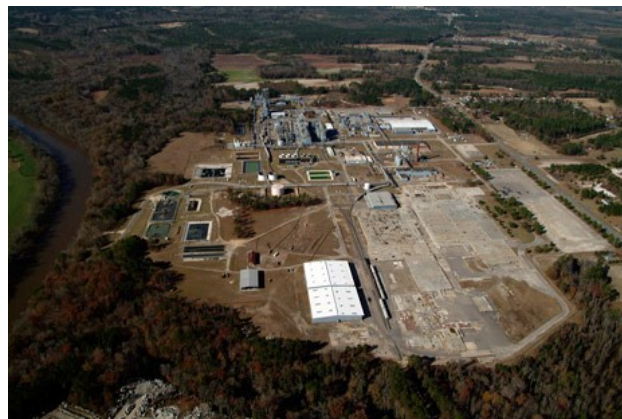
An aerial view of the Clear Path site in Fayetteville is seen here prior to construction.
