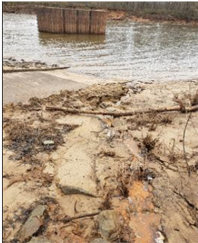
Lock and Dam Seep at boat ramp
