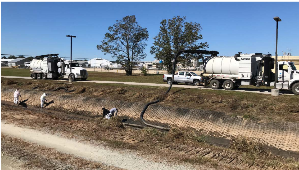
Figure 11: Sediment removal from Open Channel on October 15, 2019
