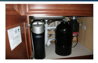
Openings on the membrane are so small that water molecules are almost the only compound that can pass through. Information on how RO systems work and their application to PFAS contamination can be found at the links at the bottom of this factsheet.
