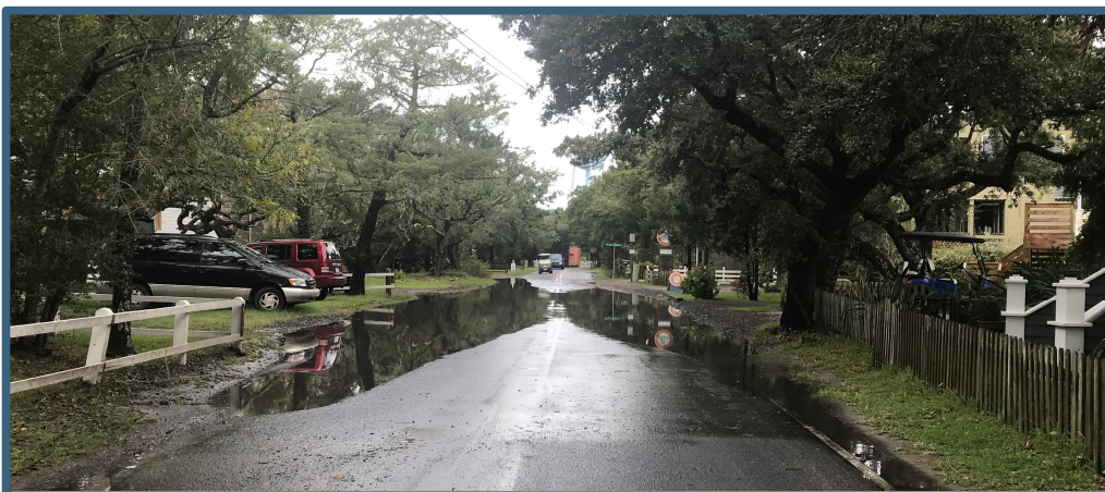
Figure 3: Back Road in Ocracoke Village following a rainstorm.
