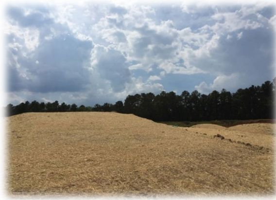
Figure 9 - Good Application of Ground Cover
