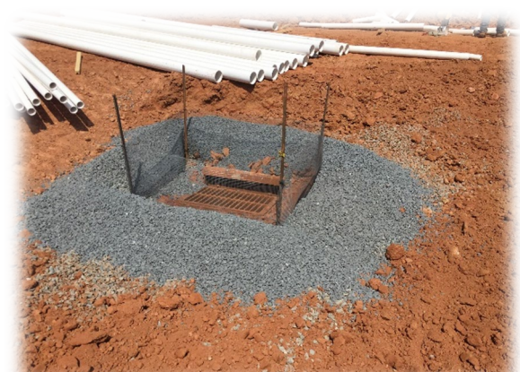
Figure 13 - Good Inlet Protection
