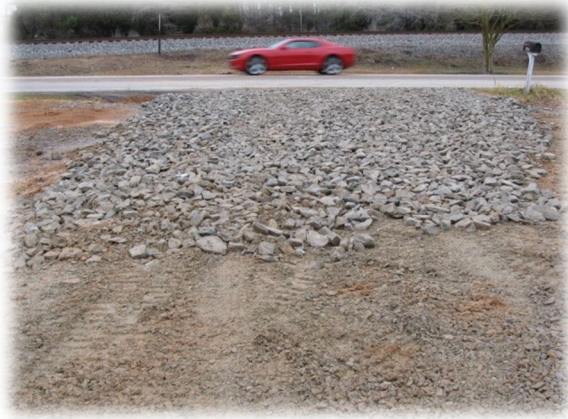
Figure 7 - Good Construction Entrance
