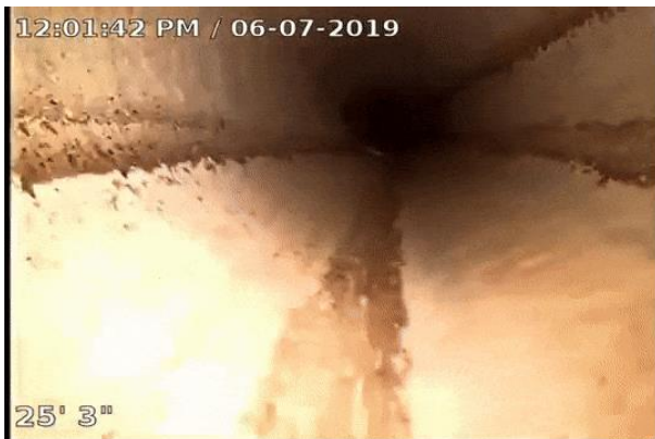
Camera inspection -Clean Pipe
