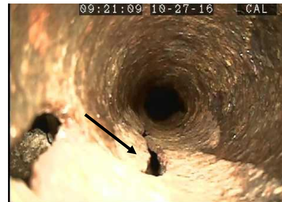
Cracked Pipe
