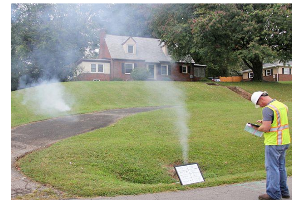
Smoke test- Leaky Pipe
