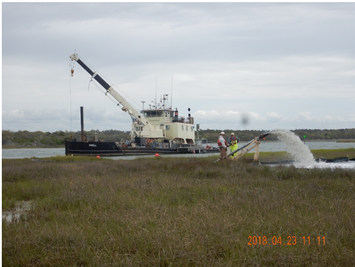
Snell pumping sediment to pond April 2018
