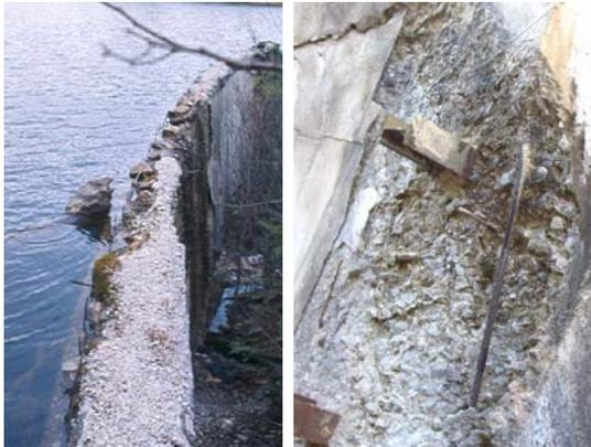
Right: Spalling Concrete.
