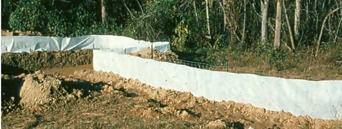
*Sediment collected by silt fence used to slow the velocity of flowing water.*
