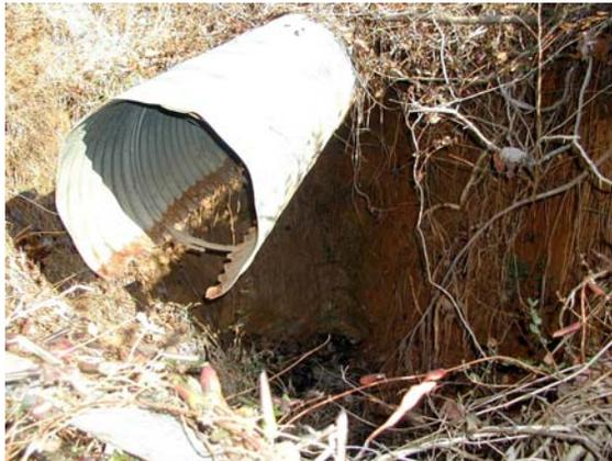
Right: Corroded pipe spillway.
