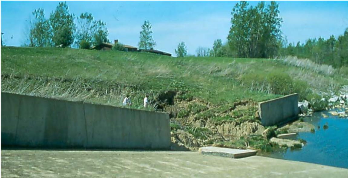
Collapse of spillway wall section.
