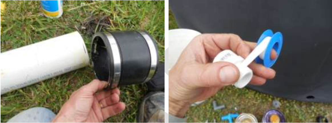
Figure 25-18. Ensure the connections are water-tight. (NCSU BAE)
