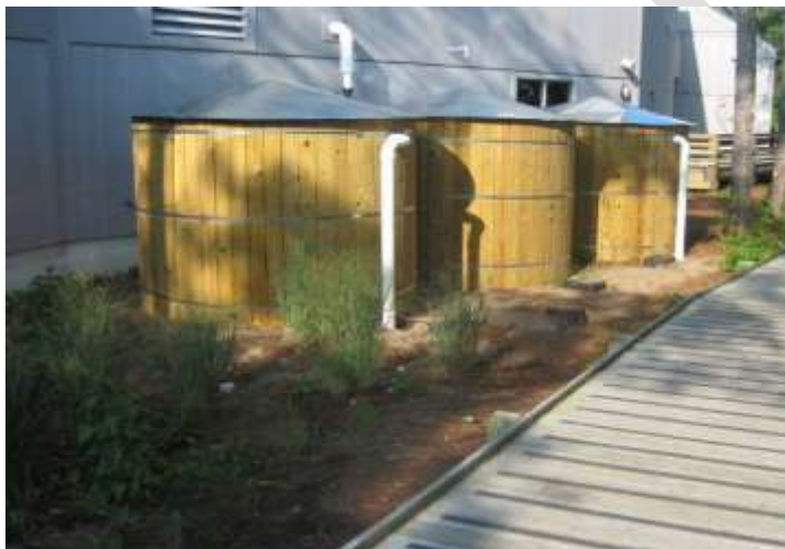
Figure 25-9. A bioretention cell adjacent to cisterns (NCSU BAE)
