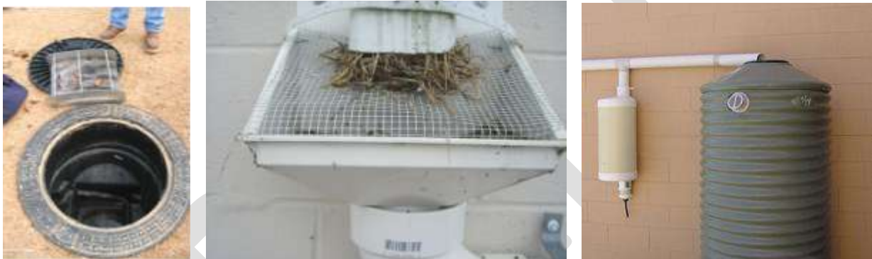
Figure 25.11. Fine filter used upstream of an underground cistern (left), gutter screen (center), downspout screen (right) (NCSU BAE left and center and UNC-CH right).
