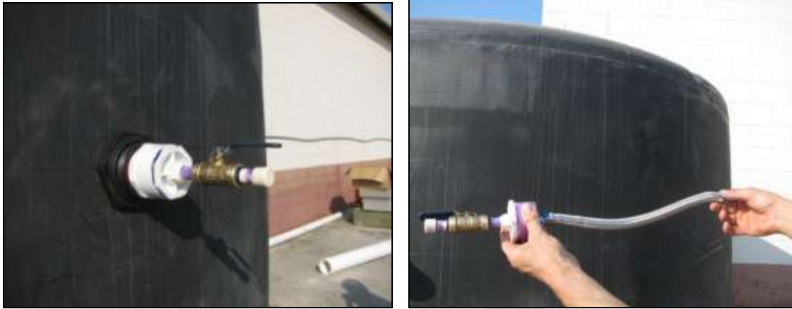
Figure 25-8. Anti-Clogging Passive Drawdown Mechanism (NCSU BAE)
