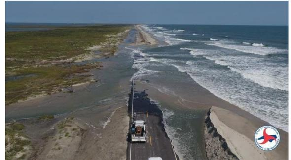
**Figure 5J- 5: NC-12 on Ocracoke Island washed out after Hurricane Dorian**
