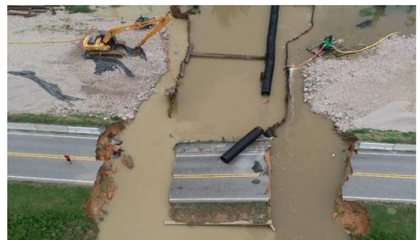
**Figure 5J-5: The Little River washed out US- 401 in northeast Wake County**
