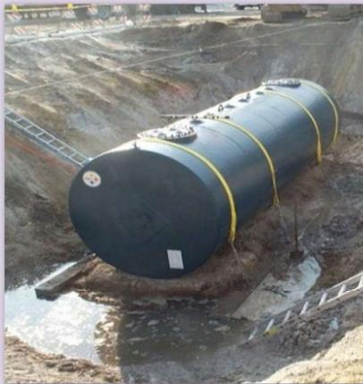
*UST with hold down straps on a concrete pad. Credit: EPA*
