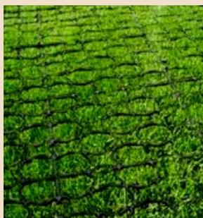
PTRG, also called geocells, consists of flexible plastic interlocking units that infiltrate water through large openings filled with aggregate or topsoil and turf grass. PTRG is well suited for emergency vehicle access over lawn areas or overflow parking. PTRG is not approved for regularly used vehicular areas such as parking lots or roadways where PICP or PC should be used.
