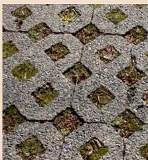
CGPs are an “older cousin” to PICPs and have significantly larger openings filled with aggregates, sand, or topsoil and turf grass for infiltration. CGPs are intended for limited vehicular traffic such as overflow parking (e.g., intermittent stadium parking), emergency access fire lanes around buildings, and median crossovers. CGP is not recommended for regularly used parking areas and for roads intended for PICP or PC.
