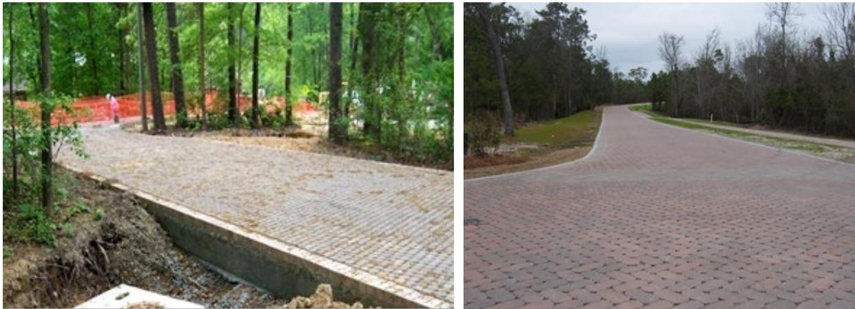
Edge restraints shall be flush with the pavement or somewhat higher than the pavement surface. Edge restraints higher than the pavement surface help keep the stormwater on the pavement and prevent stormwater run-on from clogging the permeable pavement. In addition to providing structural support, the PICP can provide an attractive edge. See Figure 6 below for examples of acceptable edge restraints.
