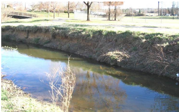
Figure 1. Streambank erosion at Burlington's City Park contributes to pollution in Little Alamance Creek.
