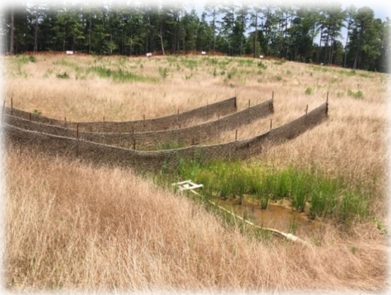
Figure 12 - Good Vegetative Stabilization
