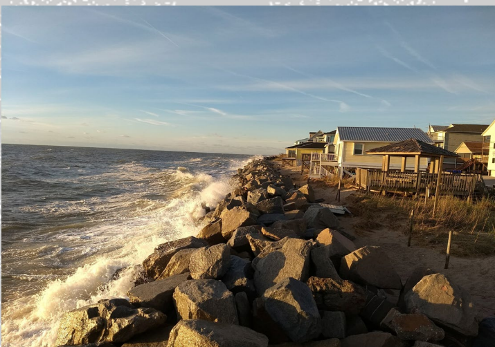
The rock vetment/embankment on the North End protects the properties behind it. These images compare the severe erosion caused by Hurricane Florence in 2018 and the beach following the nourishment project of 2019.
