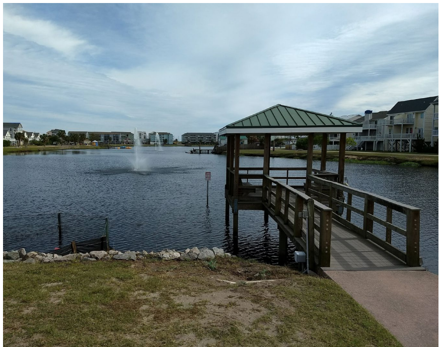
The lake was recently dredged and upfitted with larger pumps to better manage stormwater.
