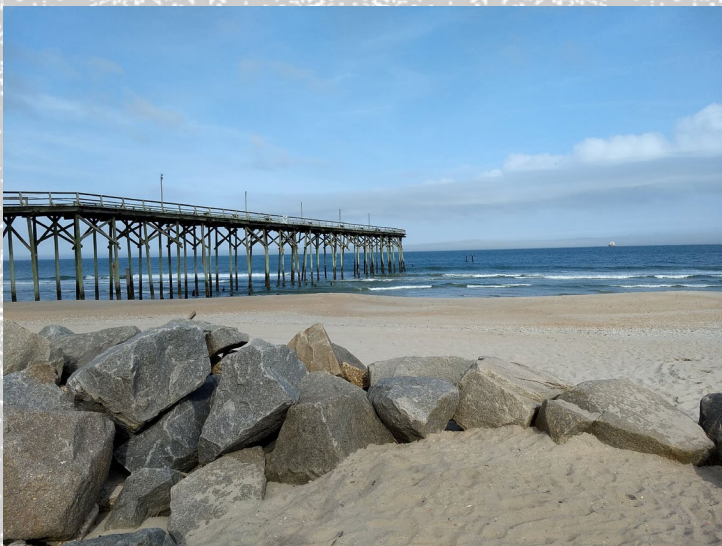
The pier on the North End.
