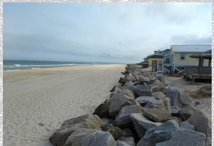
The rock vetment/embankment on the North End protects the properties behind it. These images compare the severe erosion caused by Hurricane Florence in 2018 and the beach following the nourishment project of 2019.
