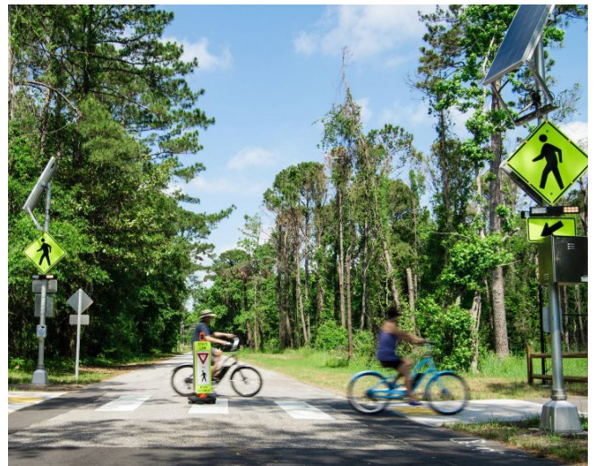
Newly installed Rectangular Rapid Flashing Beacons (RRFBs) were installed to improve pedestrian and bicycle safety and driver yielding compliance on Island Greenway crossings. (Photo credit: VisitNC)
