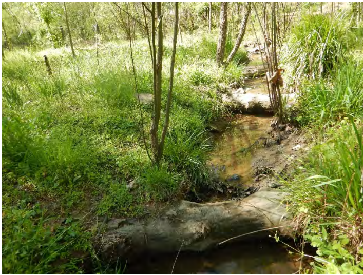
UT2 Piping Log Sills – (04/17/2020)
