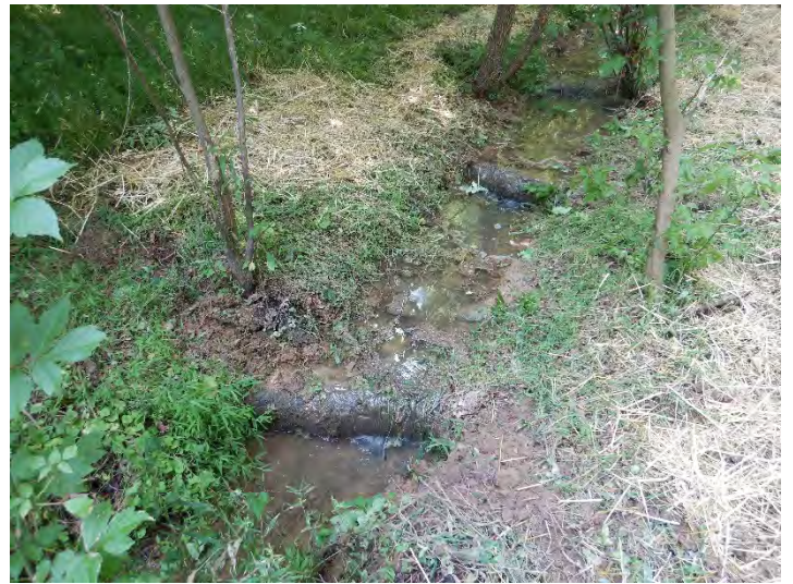
UT2 Log Sills Repaired – (07/21/2021)
