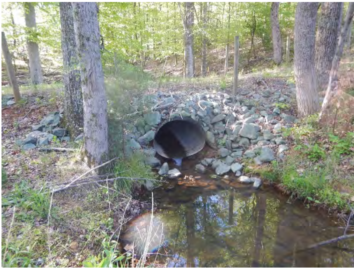
UT1A Perched Culvert – (04/17/2020)
