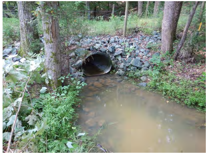
UT1A Culvert Repaired – (07/21/2021)
