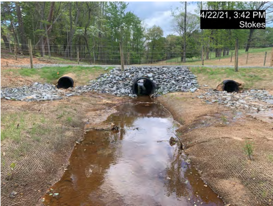
PS-9 – UT4-R1 Culvert Crossing, Upstream (MY-00)
