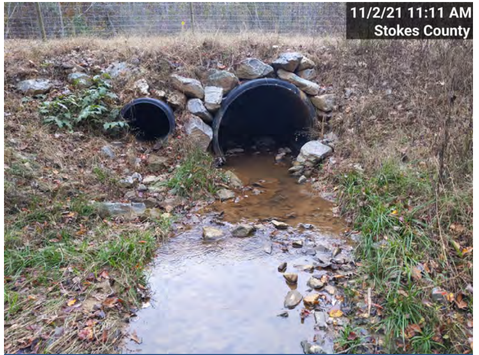
PS-6 – UT1-R2 Culvert Crossing, Upstream (MY-01)
