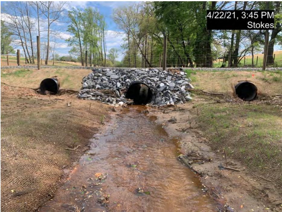
PS-9 – UT4-R1 Culvert Crossing, Downstream (MY-00)
