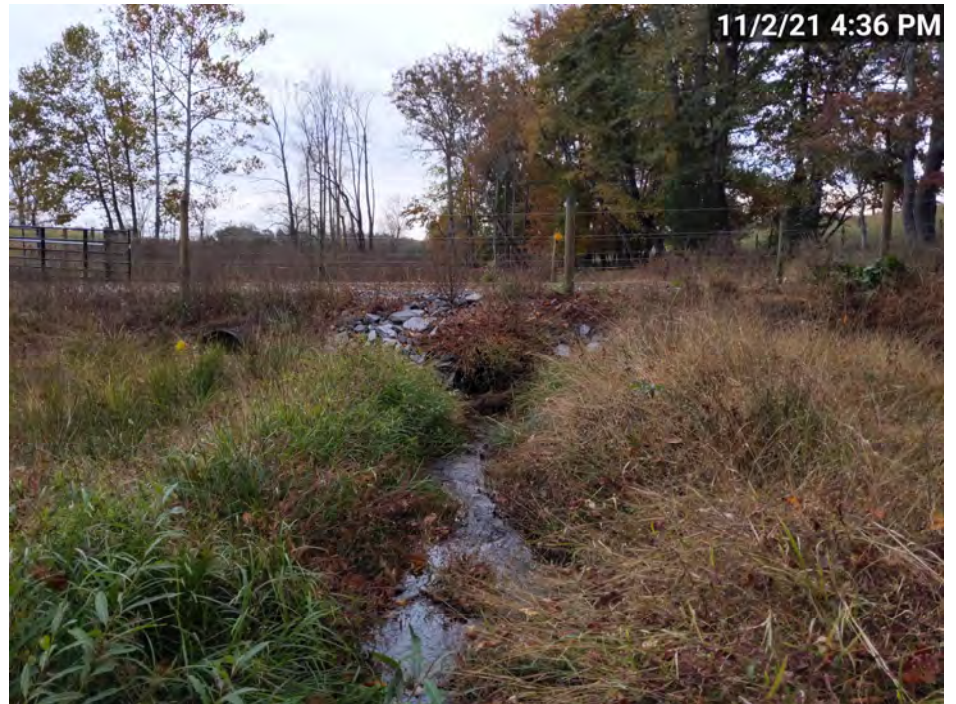
PS-9 – UT4-R1 Culvert Crossing, Downstream (MY-01)
