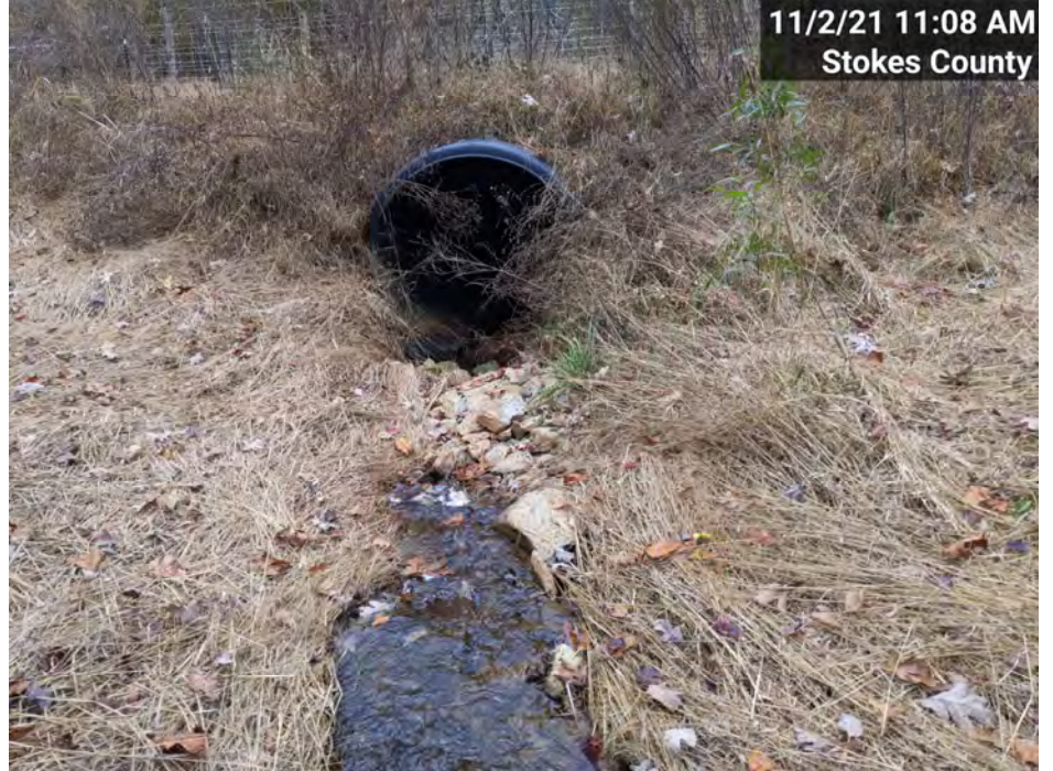
PS-6 – UT1-R2 Culvert Crossing, Downstream (MY-01)
