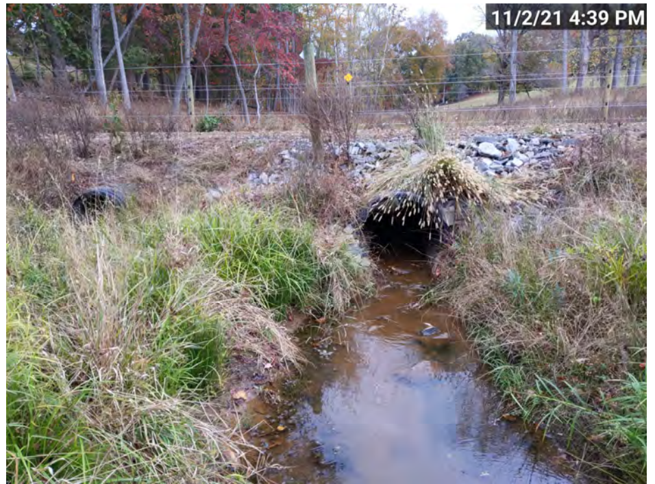
PS-9 – UT4-R1 Culvert Crossing, Upstream (MY-01)
