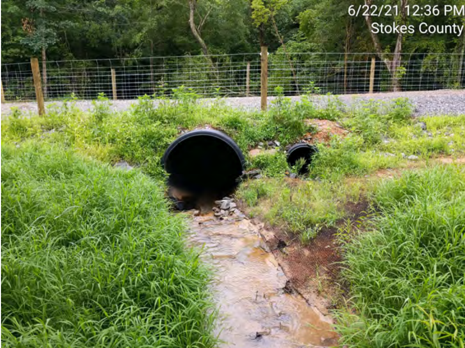
PS-6 – UT1-R2 Culvert Crossing, Downstream (MY-00)
