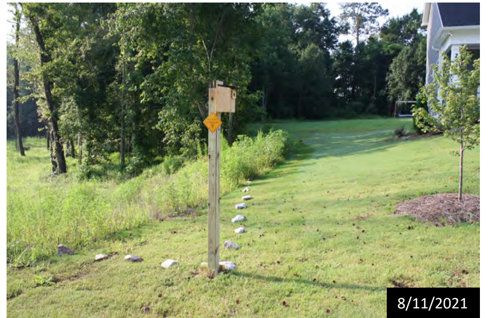
Encroachment Area 2, MS-R2, Downstream of Culvert (MY-01)
