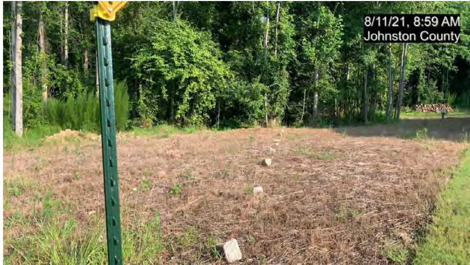
Encroachment Area 1, MS-R2, Upstream of Culvert (MY-01)
