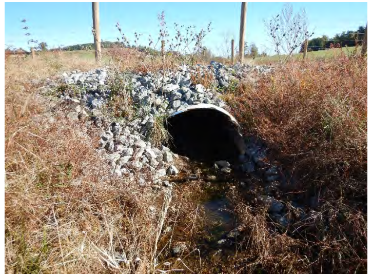
Big Bugaboo Creek R2 - Looking Downstream (10/27/2021)
