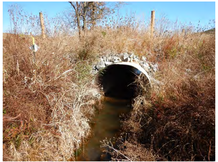
Big Bugaboo Creek R3 - Looking Downstream (10/27/2021)
