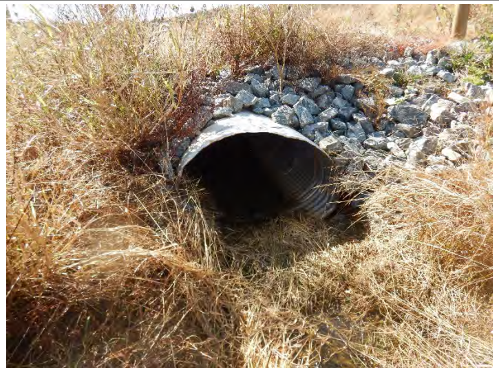
UT2 R5 - Looking Downstream (10/27/2021)
