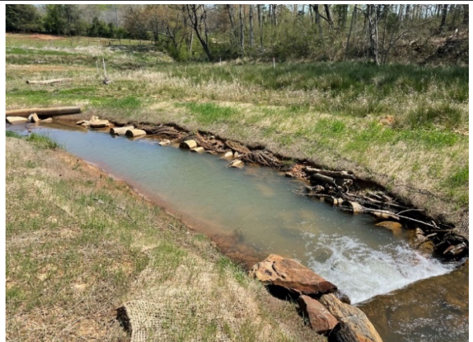
Post-Repair – STA 113+80 Downstream; Right Bank Brush Toe Repaired (04/07/2021)
