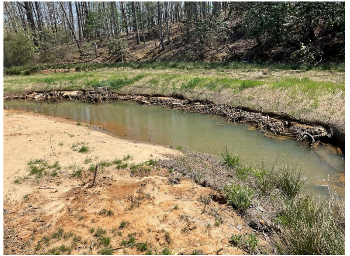
Post-Repair - STA 112+00 Downstream; Repaired Brush Toe and Added Geo-Lift (04/07/2021)
