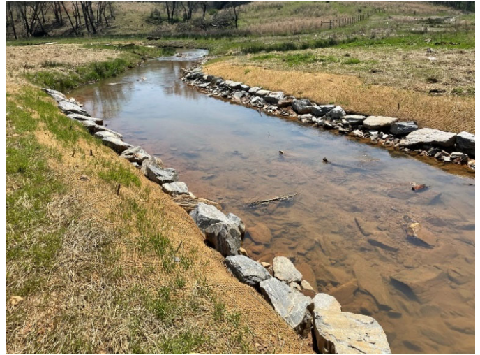
Post-Repair – STA 150+30 Downstream; Right and Left Banks Regraded and Matted (04/07/2021)
