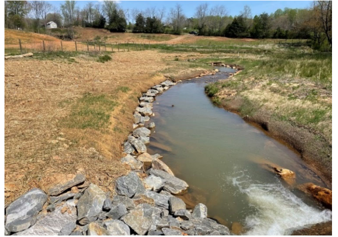
Post-Repair – STA 113+00 Downstream; Repaired Brush Toe Along Left Bank; Added a Geolift, Boulder Toe and Floodplain Outlet (04/07/2021)
