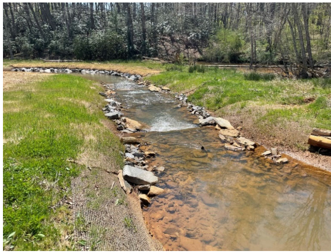
Post-Repair – STA 105+85 Downstream; Rebuilt Riffle and Regraded and Matted Left Bank (04/07/2021)
