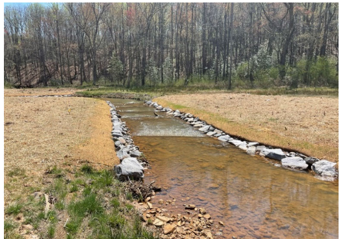
Post-Repair – STA 163+70 Downstream; Right and Left Banks Regraded and Matted (04/07/2021)
