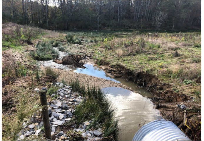
Pre-Repair – STA 211+50 Downstream; Erosion Along Right Bank (11/02/2020)
