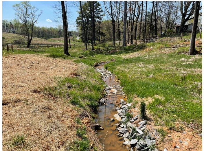
Post-Repair – STA 405+40 – 405+65 Downstream; Added Riffle Material (04/07/2021)
