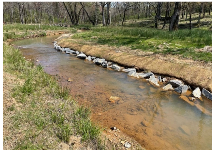
Post-Repair – STA 156+35 Downstream; Right Bank Regraded and Matted (04/07/2021)
