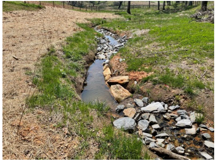
Post-Repair – STA 404+90 – 405+30 Downstream; Added Riffle Material (04/07/2021)
