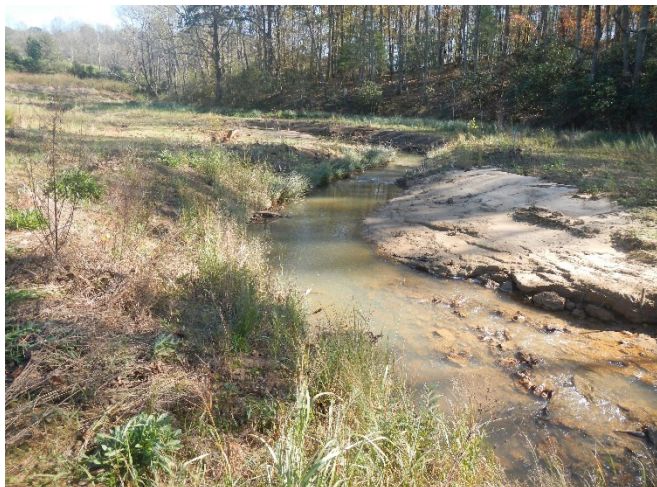
Pre-Repair – STA 111+25 Downstream; Scour on Right Bank from Point Bar into Riffle (11/03/2020)
