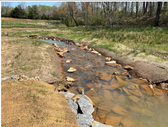
Post-Repair – STA 113+40 Downstream; Repaired Riffle and Scraped and Re-Matted Banks (04/07/2021)
