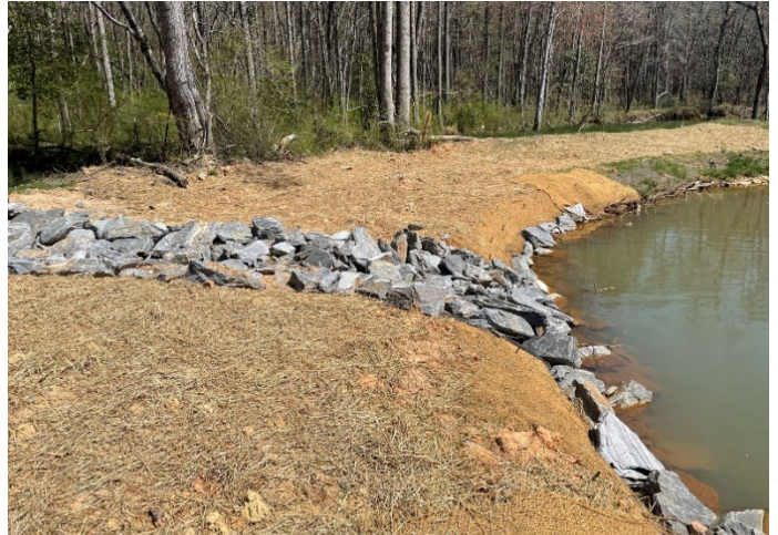
Post-Repair – STA 163+00 Downstream; Installed Rock-Lined Swale and Outlet; Repaired Brush Toe & Added Geolift Along Left Bank (04/07/2021); Regraded and Matted Right Bank (Not Shown)
