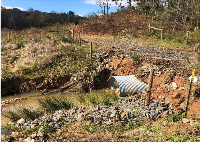
Pre-Repair – STA 211+50 From Left Bank; Erosion along Downstream Side of Crossing and Around Culvert (11/02/2020)
