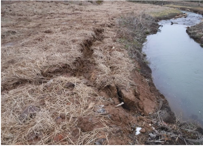
Pre-Repair – STA 113+00 Downstream; After the November Repair a Floodplain Seep Created Erosion Behind Brush Toe and Outlet (12/30/2020)
