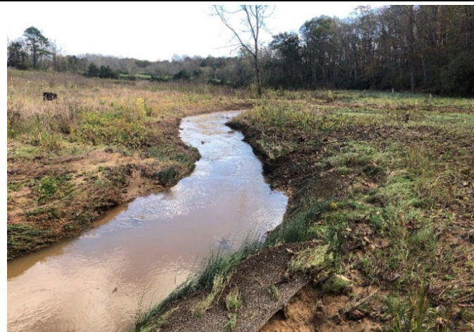
Pre-Repair – STA 107+00 Downstream; Erosion Along Right and Left Banks (11/02/2020)
