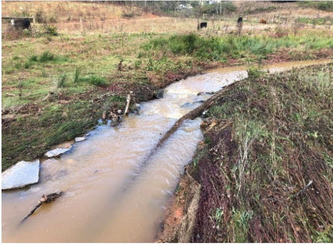
Pre-Repair – STA 114+20 Downstream; Riffle Scour (11/02/2020)
