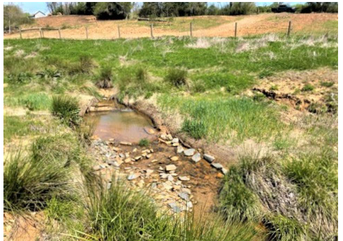
Post-Repair – STA 212+30 Upstream; Left Bank Regraded and Matted (04/07/2021)
