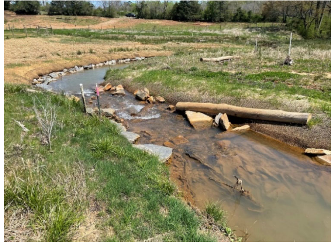
Post-Repair – STA 114+20 Downstream; Repaired Riffle (04/07/2021)
