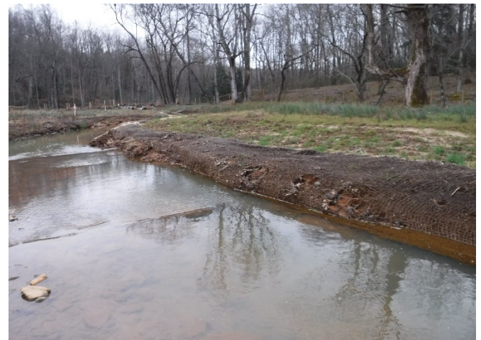
Pre-Repair – STA 156+35 Downstream; Erosion Along Right Bank (10/30/2020)
