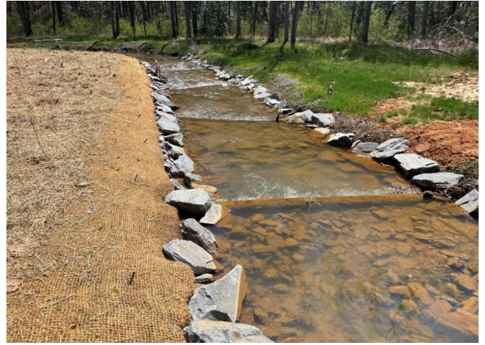
Post-Repair – STA 160+65 Downstream; Left Bank Regraded and Matted (04/07/2021)
