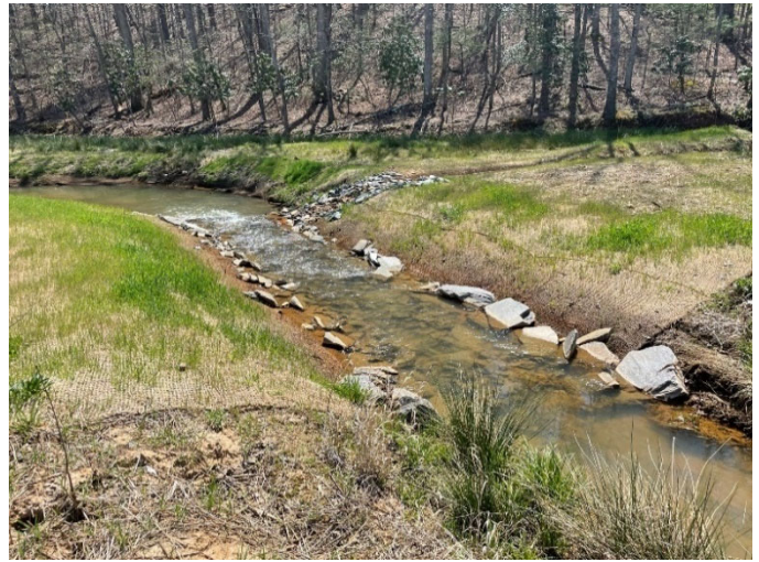
Post-Repair – STA 109+80 Downstream; Rebuilt Riffle, Reset Log Sill, and Moved Floodplain Outlet Upstream (04/07/2021)
