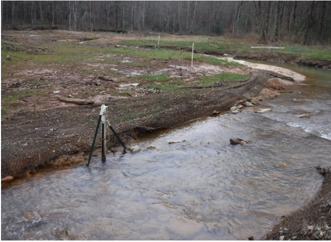
Pre-Repair – STA 160+65 Downstream; Erosion Along Left Bank (12.30.20)
