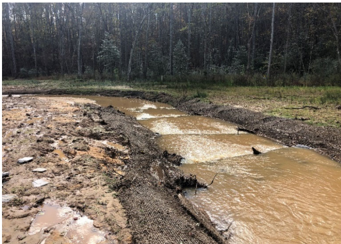
Pre-Repair – STA 163+70 Downstream; Erosion Along Right and Left Banks (11/02/2020)
