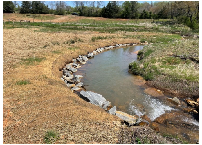
Post-Repair – STA 114+50 Downstream; Replaced Brush Toe with Geo-Lift and Boulder Toe (04/07/2021)
