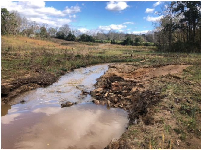
Pre-Repair – STA 110+65 Downstream; Scour Pocket Along Right Bank and Displacement of Riffle Material (11/02/2020)
