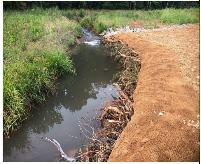
Post-Repair – A2 113+25 A4 (08/16/2021)
