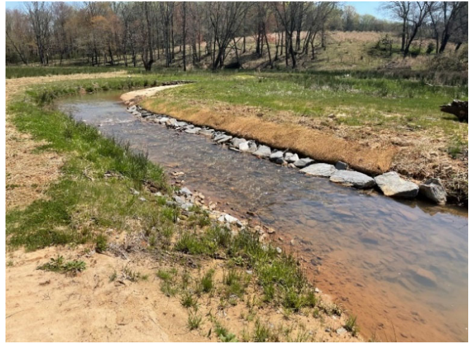
Post-Repair – STA 152+10 Downstream; Right Bank Regraded and Matted (04/07/2021)
