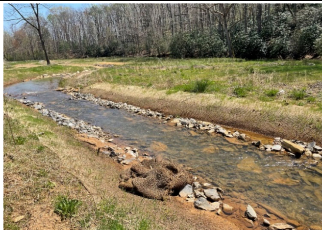
Post-Repair – STA 107+00 Downstream; Right and Left Banks Regraded and Matted (04/07/2021)
