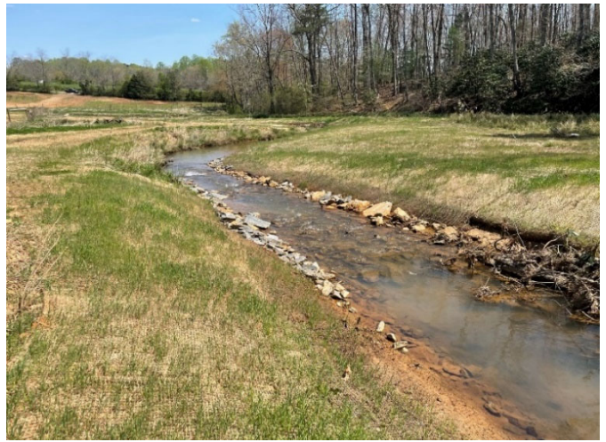
Post-Repair – STA 110+65 Downstream; Extended Brush Toe Along Right Bank and Rebuilt Riffle (04/07/2021)
