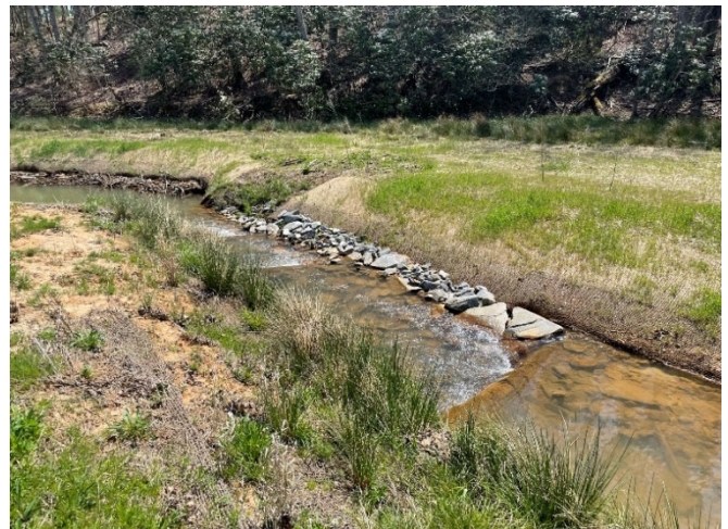
Post-Repair – STA 111+70 Downstream; Right Bank Regraded and Matted (04/07/2021)
