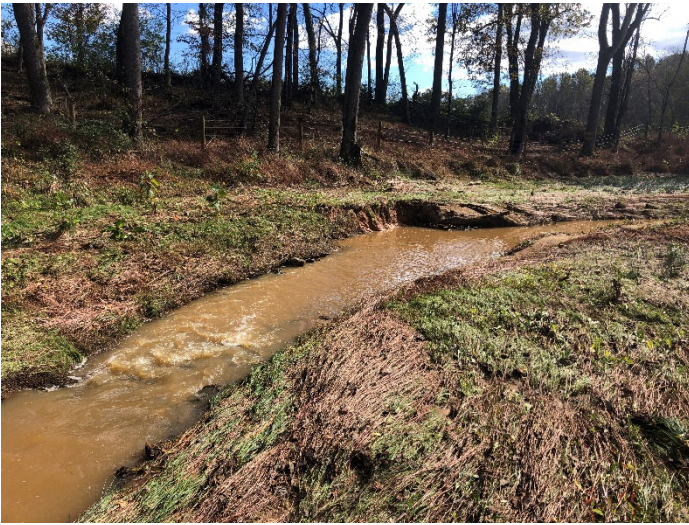
Pre-Repair – STA 102+00 Downstream; Erosion Along Left Bank and Brush Toe (11/02/2020)
