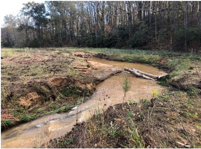
Pre-Repair – STA 109+80 Downstream; Riffle Failure, Dislodged Log Sill, and Erosion Along Point Bar (11/02/2020)
