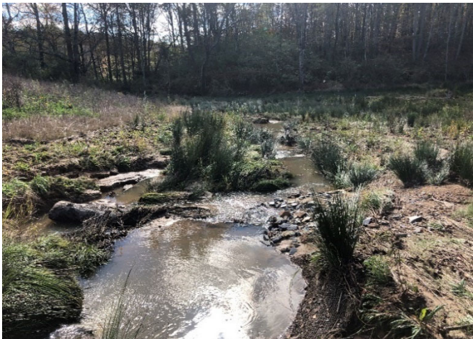
Pre-Repair – STA 212+30 Downstream; Erosion Along Left Bank Causing Channel Migration (11/02/2020)
