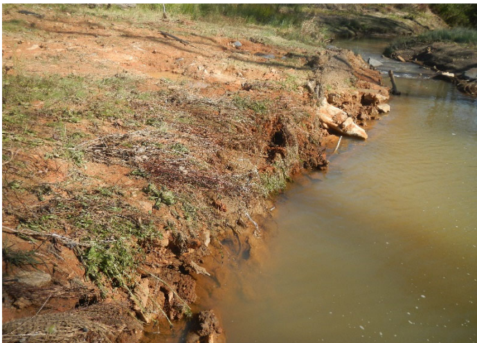
Pre-Repair – STA 115+35 Downstream; Erosion Along Right Bank (11/02/2020)
