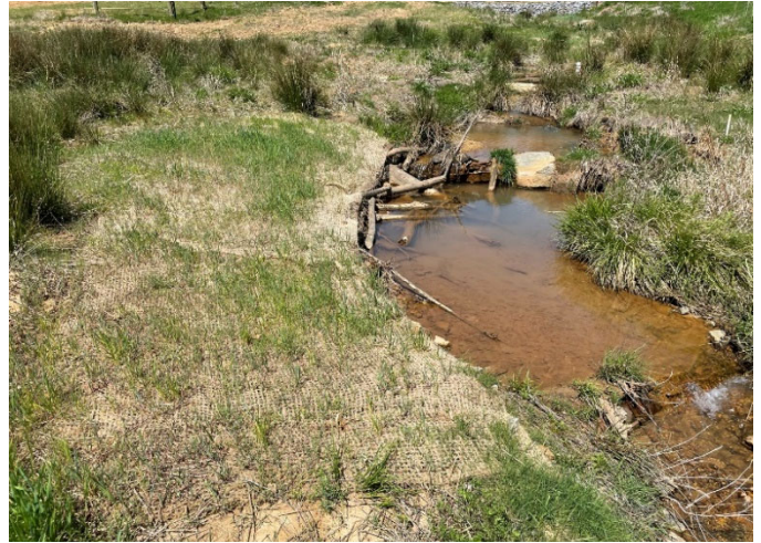
Post-Repair – STA 212+80 Upstream; Installed Brush Toe Along Right Bank (04/07/2021)
