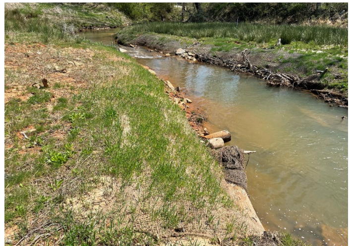
Post-Repair – STA 115+35 Downstream; Regraded and Installed Brush Toe along Right Bank (04/07/2021)
