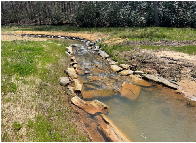
Post-Repair – STA 107+90 Downstream; Right and Left Banks Regraded and Matted (04/07/2021)
