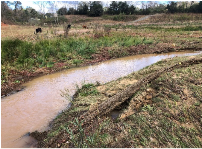
Pre-Repair – STA 114+65 Downstream; Erosion Along Left Bank and Brush Toe (11/02/2020)
