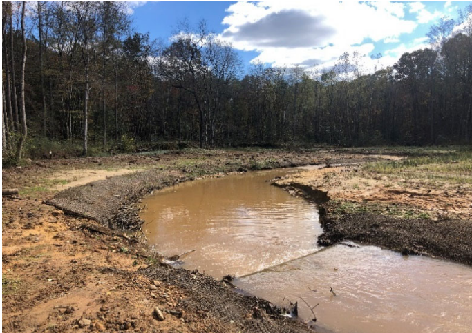
Pre-Repair – STA 163+00 Downstream; Left Bank Erosion from Floodplain Discharge and Erosion Along Right Bank (11/02/2020)
