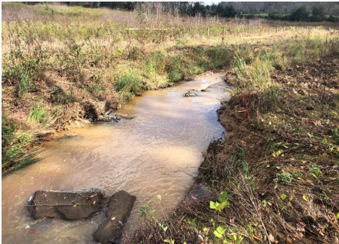
Pre-Repair – STA 108+70 Downstream; Loss of Riffle Material and Dislodged Log Sill (11/02/2020)
