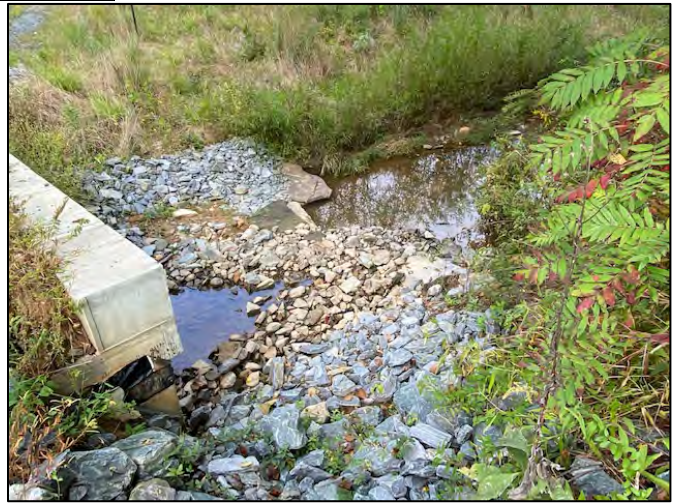
Repaired boulder sill – 7/23/21
