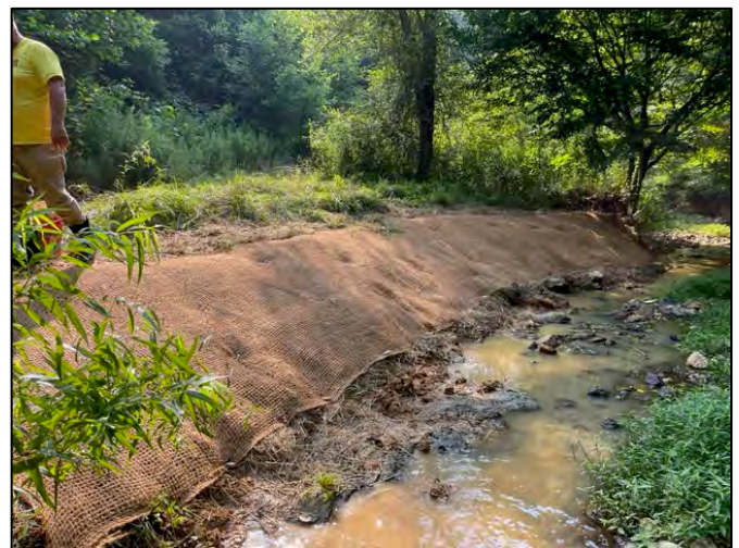
STA 61+00 after repair – 7/23/21
