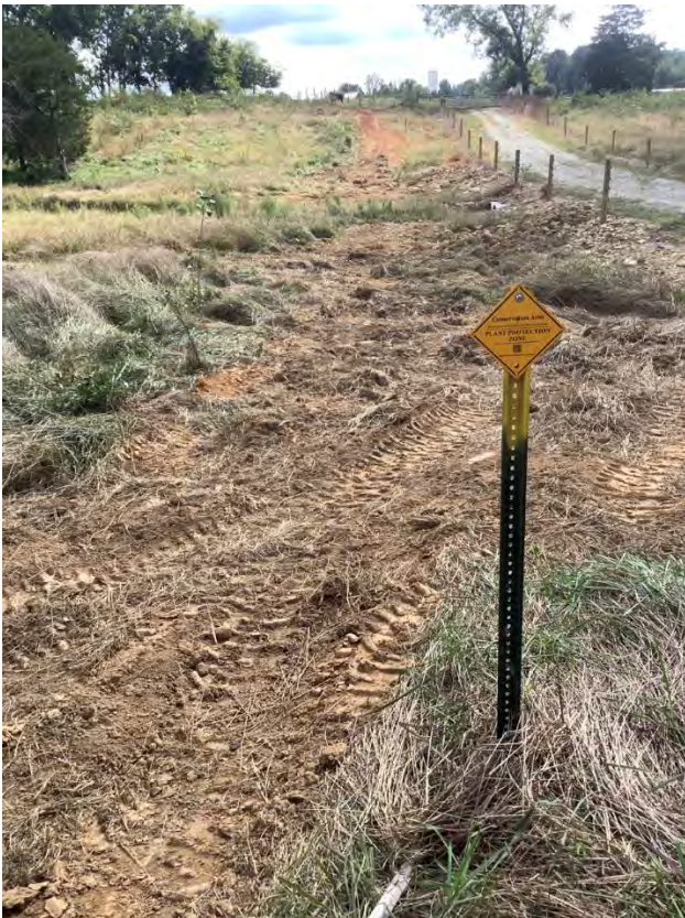
Perry Branch Reach 4 – CE Encroachment (10/04/2021)
