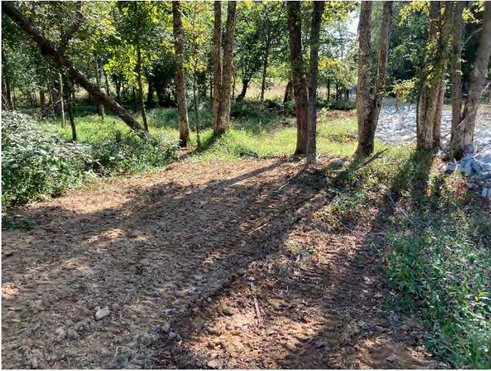
Perry Branch Reach 2 – CE Encroachment (10/04/2021)
