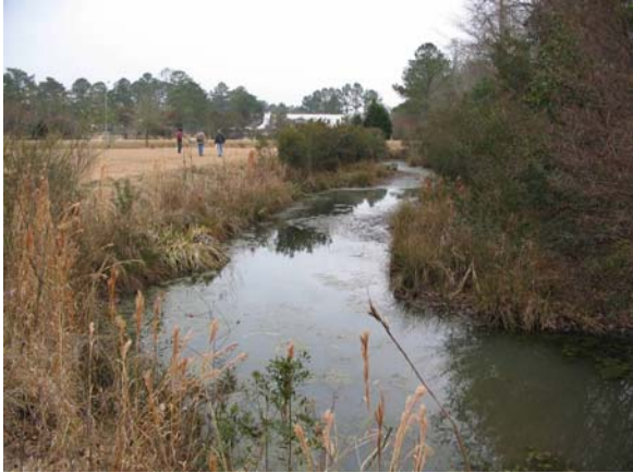
Figure 1. River Bend wetland before being resized and reconstructed.
