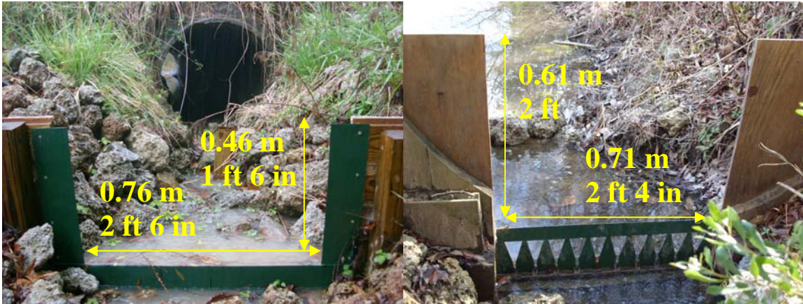
Figure 12. From left: inflow and outflow weirs.
