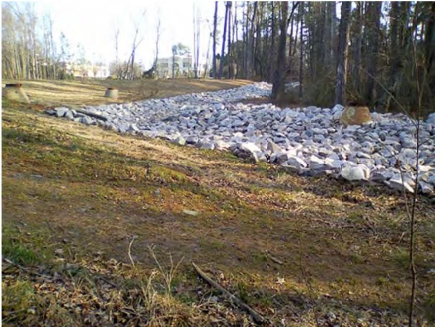
Figure 6. Emergency spillway
