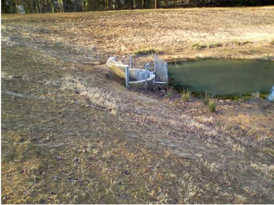
Figure 5. Primary outlet structure and trash rack
