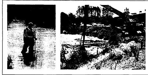
Figure 2. Inspection (A) of sediment depth and cleaning or "dipping" (B) of forebays. A long boom on the excavator is sometimes essential to access sediment collected in the middle of the forebay.
