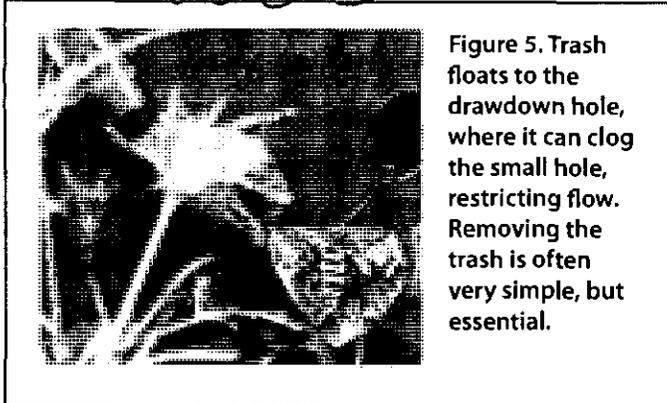
Figure 5. Trash floats to the drawdown hole, where it can clog the small hole, restricting flow. Removing the trash is often very simple, but essential.
