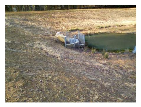
Figure 5. Primary outlet structure and trash rack
