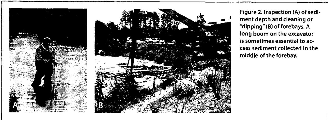
Figure 2. Inspection (A) of sediment depth and cleaning or "dipping" (B) of forebays. A long boom on the excavator is sometimes essential to access sediment collected in the middle of the forebay.
