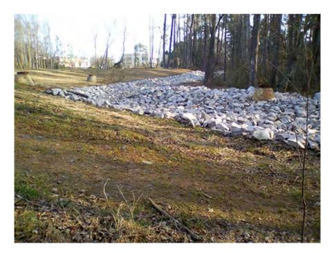
Figure 6. Emergency spillway
