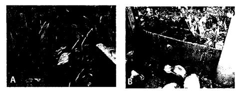
Figure 4. A small orifice allows slow release of captured stormwater (A), but can easily clog due to its size. A clogged orifice can affect plant communities inside the wetland or wet pond (B).
