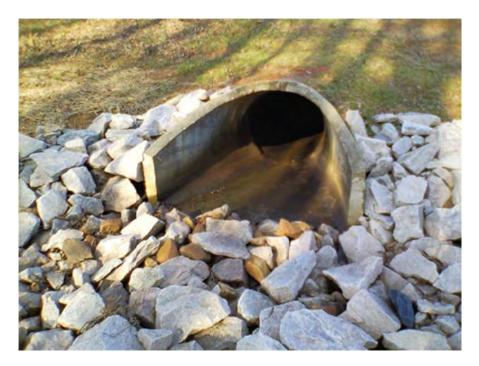
Figure 7. Primary wetland outlet pipe
