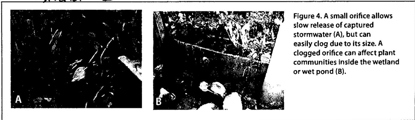
Figure 4. A small orifice allows slow release of captured stormwater (A), but can easily clog due to its size. A clogged orifice can affect plant communities inside the wetland or wet pond (B).
