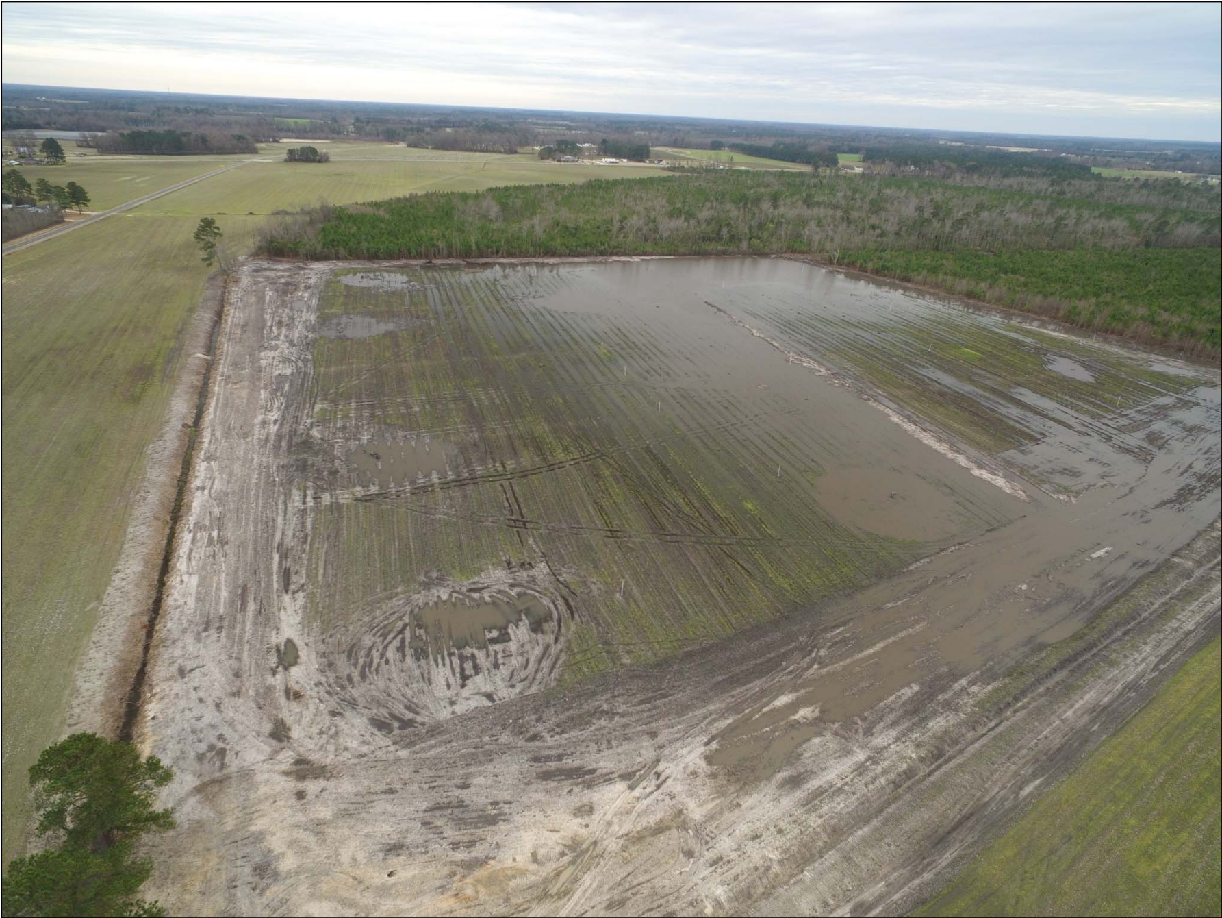
Looking south at W1 (1/31/2020)
