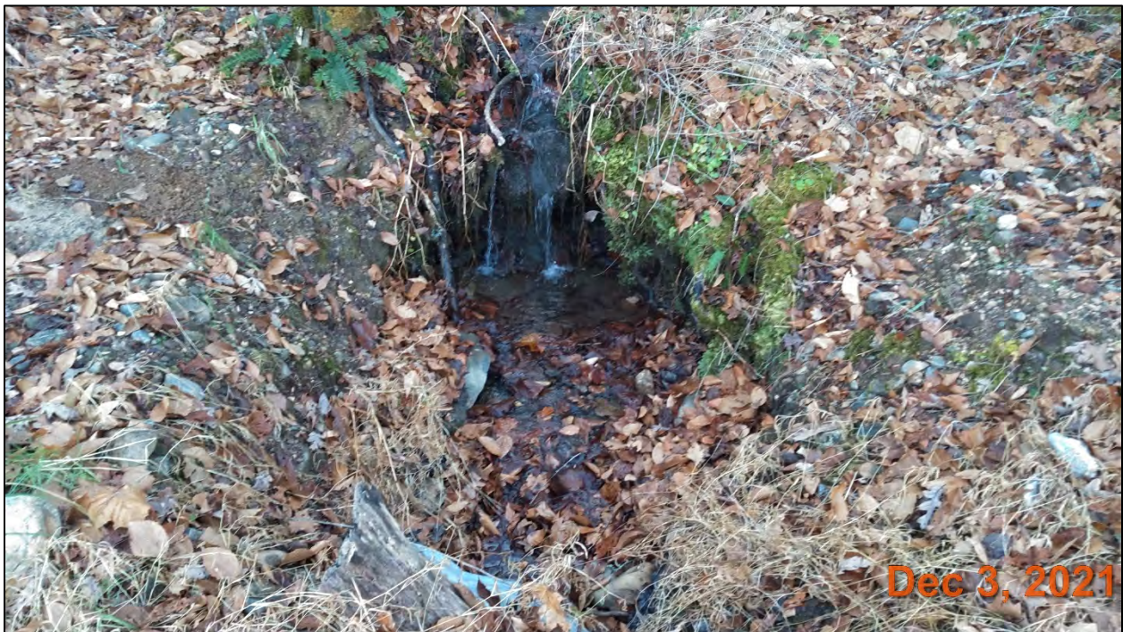
Photo point #1 supplemental, facing stormwater control measure along Reach 1A boundary.
