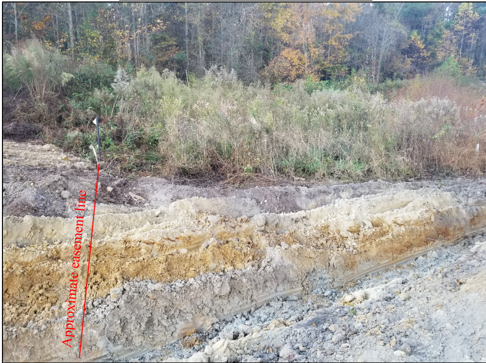
Photo 1 – View of encroachment looking along the easement line
