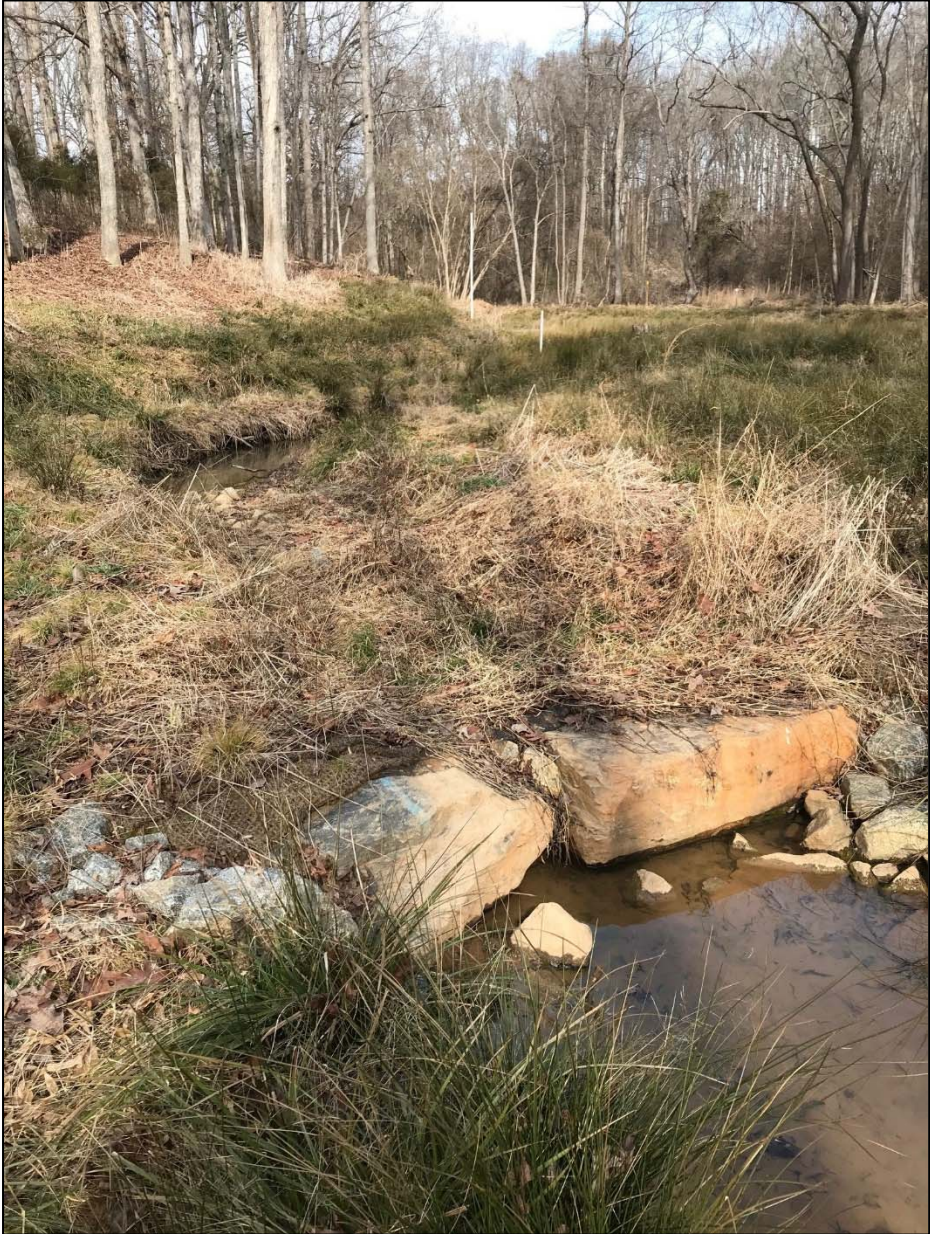
UTWB-1 Station 12+40 piping rock sill (2/3/2022)
