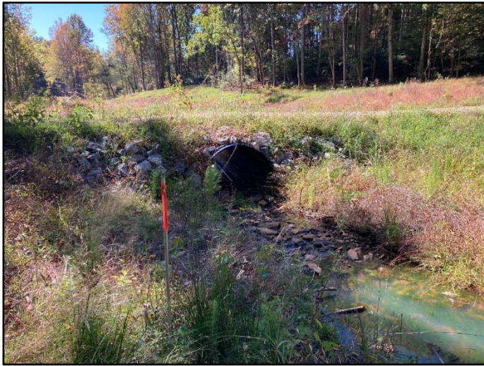
Photo Station 5 Crossing on UTWB-2 looking downstream
