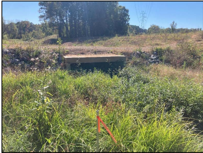
Photo Station 11 Crossing on UTWB-3 looking downstream
