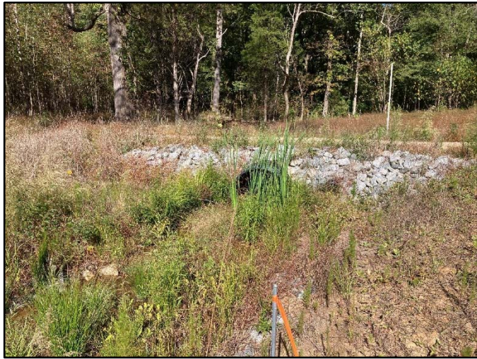
Photo Station 9 Crossing on UT2-2 looking upstream
