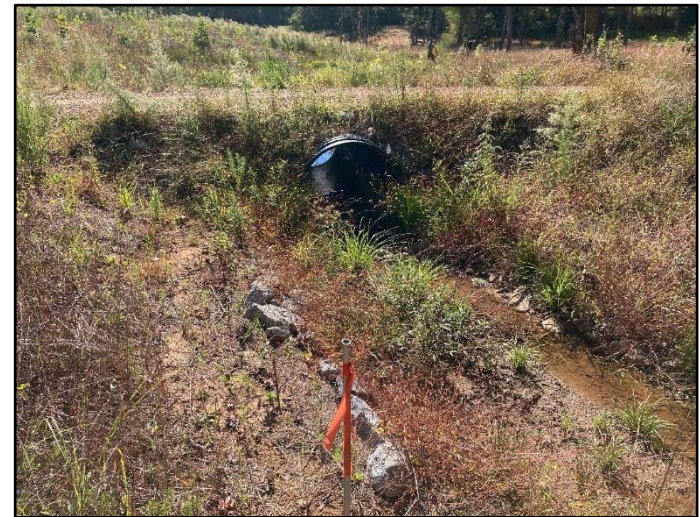
Photo Station 8 Crossing on UT2-2 looking downstream
