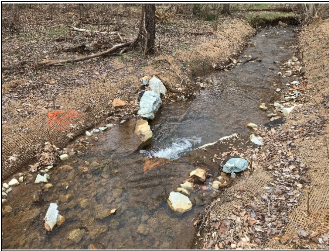
PP-27: Reach 3, view downstream, Station 14+00
