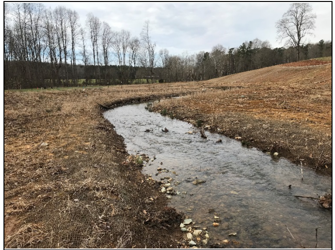
PP-2: Reach 1, view downstream, Station 11+50
