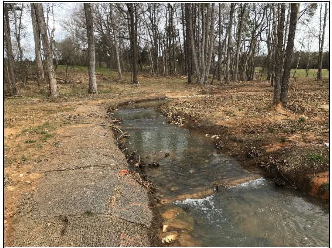
PP-10: Reach 1, view upstream, Station 27+50
