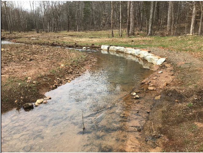
PP-13: Reach 1, view downstream, Station 30+50
