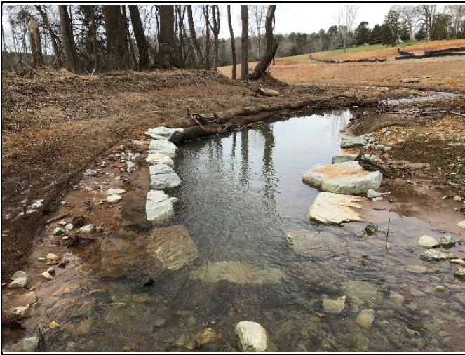
PP-1: Reach 1, view downstream, Station 10+00
