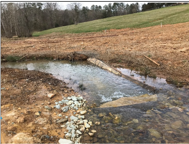
PP-5: Reach 1, view downstream, Station 16+50
