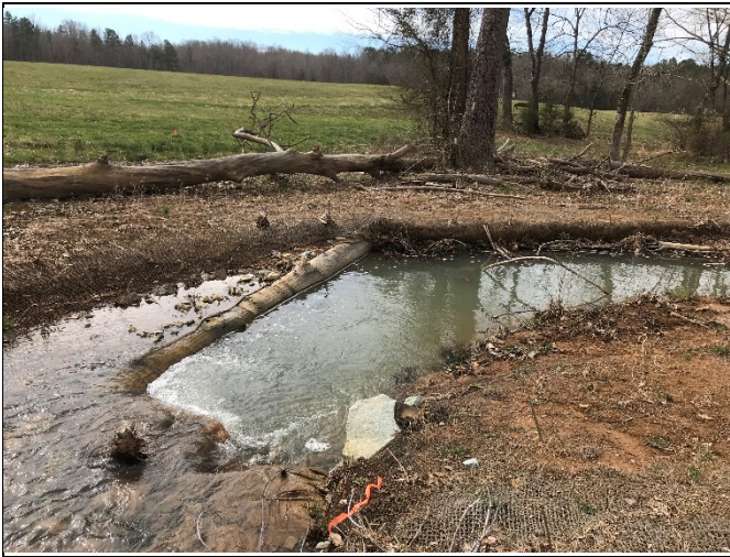
PP-7: Reach 1, view downstream, Station 21+50
