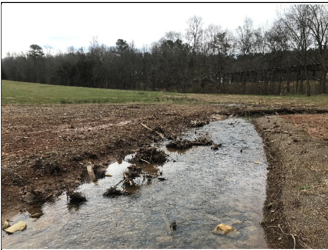
PP-11: Reach 1, view downstream, Station 29+00
