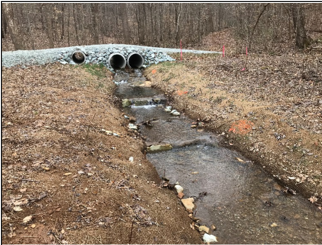
PP-23: Reach 3, view upstream, Station 10+50
