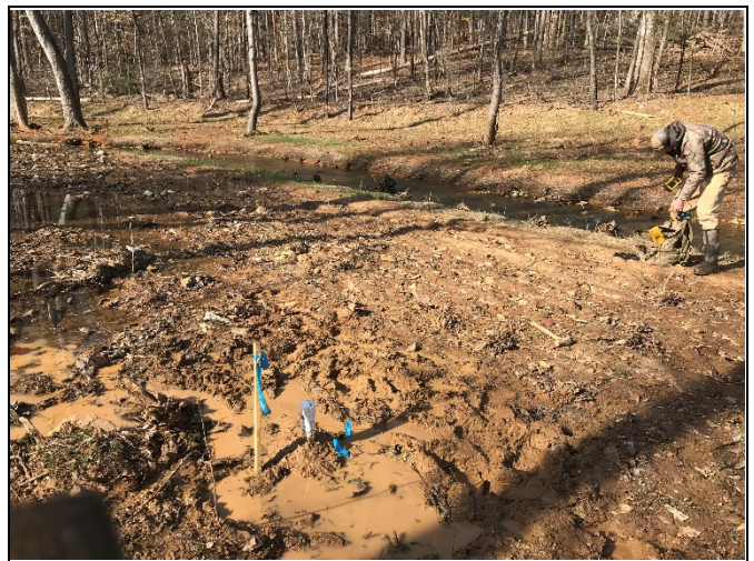
Monitoring Well #3, Reach 1, Station 36+25
