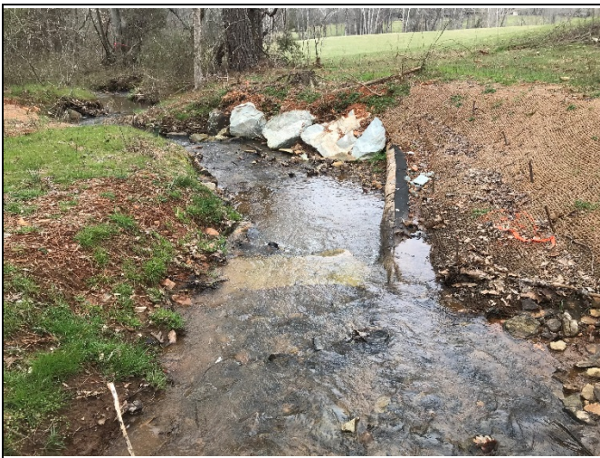
PP-29: Reach 3, view downstream, Station 18+25
