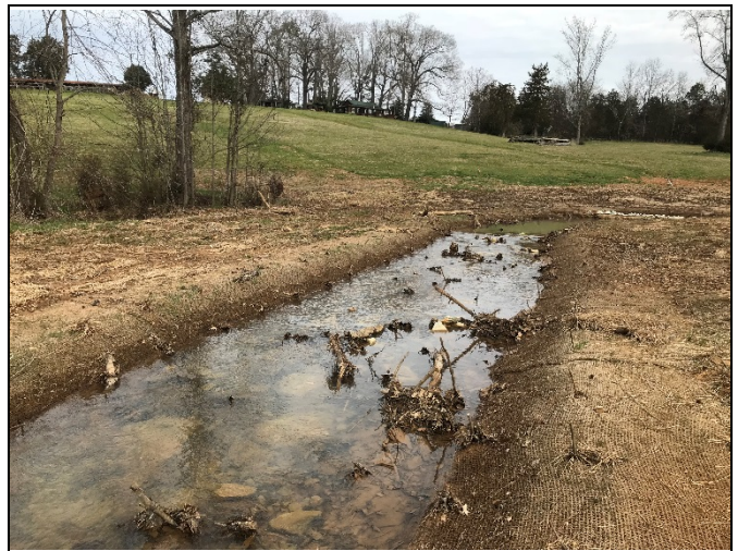
PP-6: Reach 1, view upstream, Station 19+50
