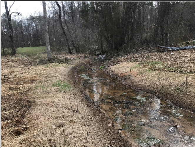
PP-21: Reach 2, view upstream, Station 15+50
