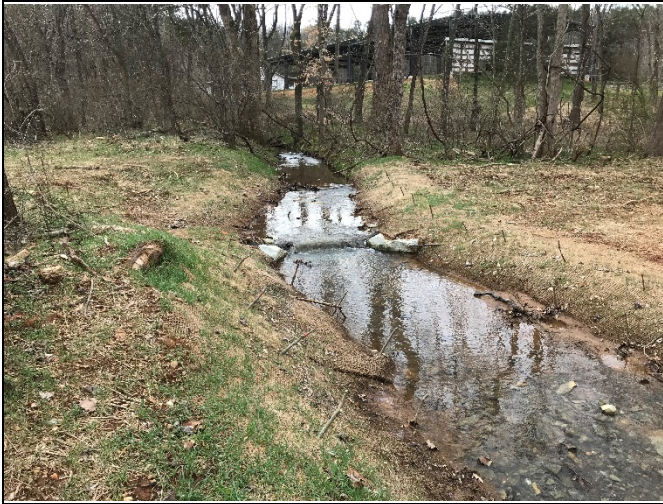
PP-31: Reach 3, view upstream, Station 25+50
