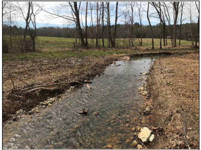
PP-8: Reach 1, view downstream, Station 23+00
