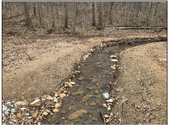
PP-24: Reach 3, view downstream, Station 10+75
