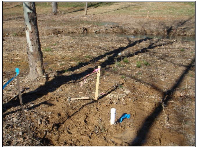
Monitoring Well #1, Reach 1, Station 20+75
