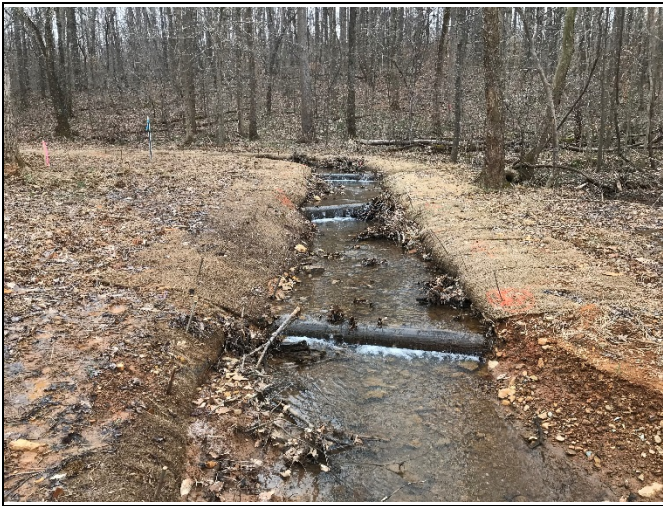
PP-25: Reach R3, view upstream, Station 11+75
