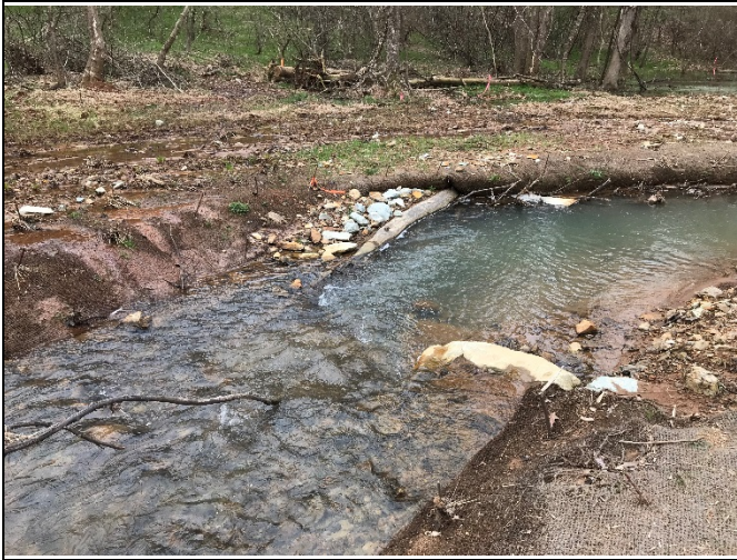
PP-19: Reach 1, view downstream, Station 39+75
