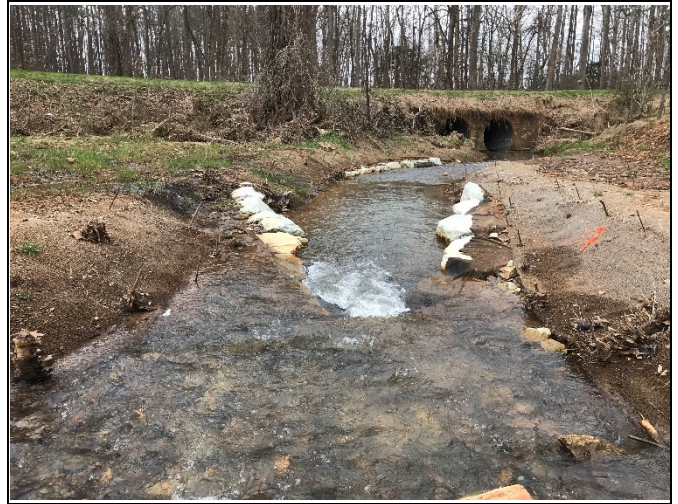
PP-20: Reach 1, view downstream, Station 41+00
