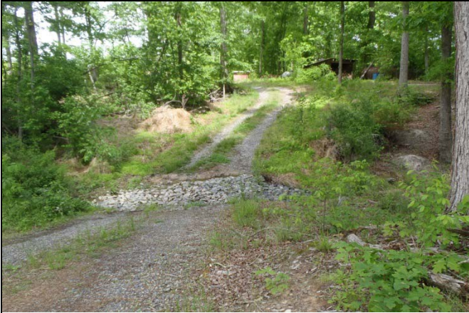
Existing ford crossing on lower Reach R3 (5/8/2013)
