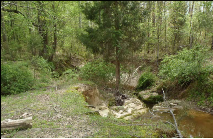
View looking at downstream end of project. Reach R1 is incised but has reached bedrock (4/16/2013)
