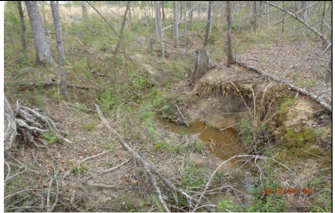
Eroding right bank along the middle Reach R3 (4/16/2013)
