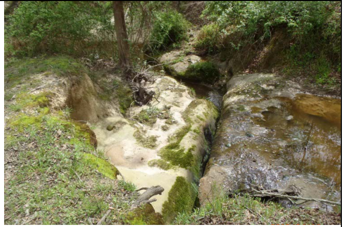
Close up of bedrock grade control at lower end of Reach R1 (4/16/2013)
