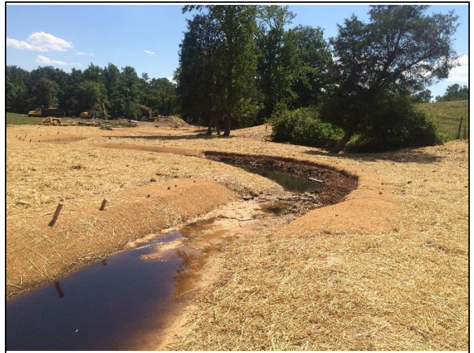
Reach 2, view downstream at Station 34+30
