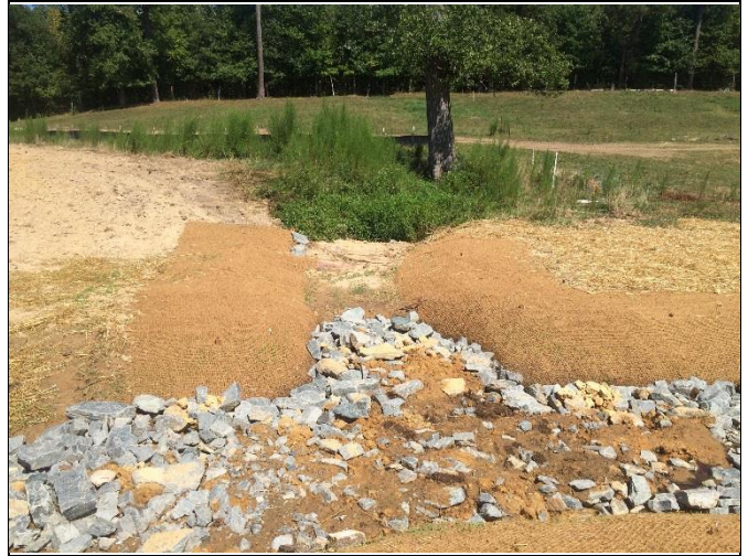
Reach 2, view of drainage on left bank at Station 32+90
