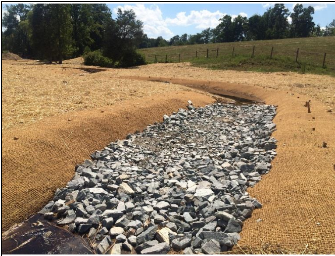
Reach 2, view downstream at Station 33+25
