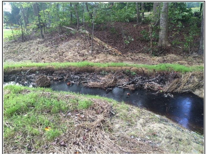
Reach 5, view downstream at Station 32+50
