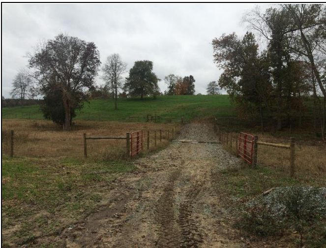
Reach 2, view of crossing at Station 27+75
