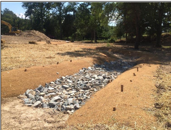
Reach 2, view downstream at Station 36+90
