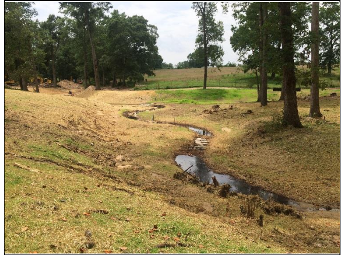
Reach 4, view downstream at Station 12+25
