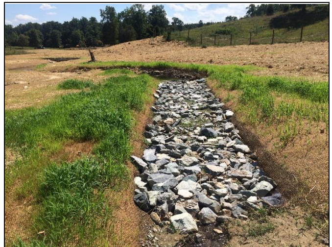
Reach 2, view downstream at Station 30+20
