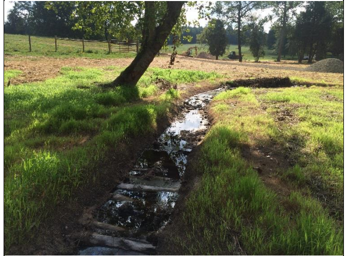
Reach 5, view downstream at Station 33+75
