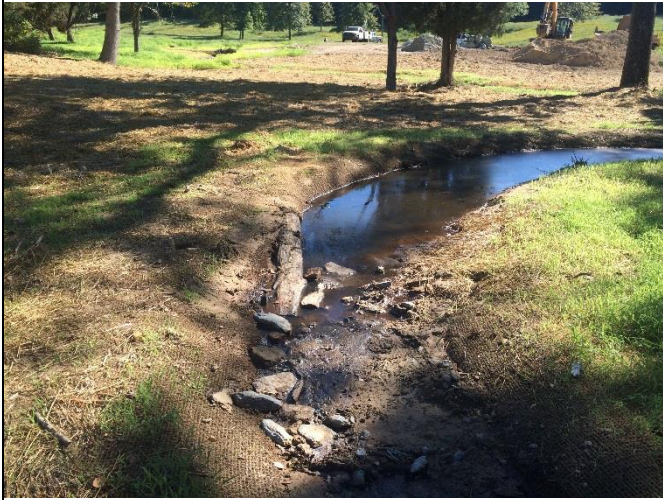
Reach 5, view downstream at Station 37+30
