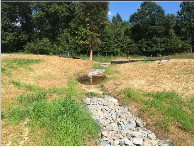
Reach T1, view upstream at Station 11+75
