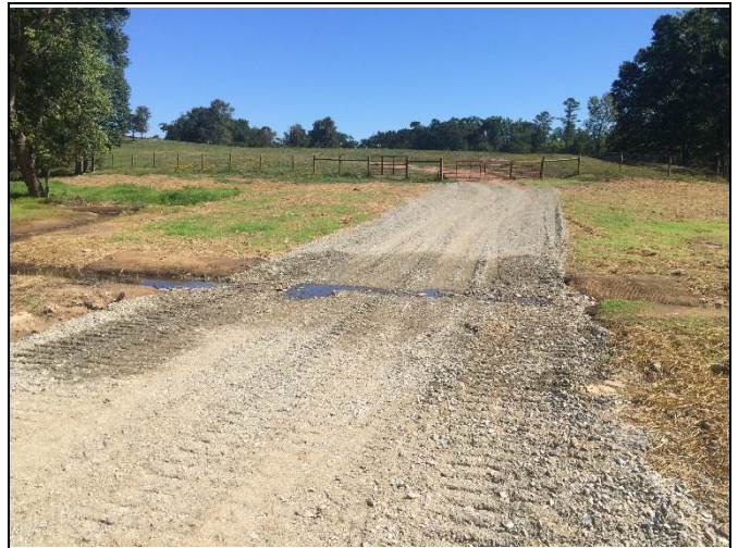
Reach 5, Rock Crossing at Station 35+00
