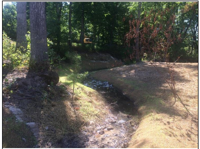
Reach 3, view downstream, Station 16+25
