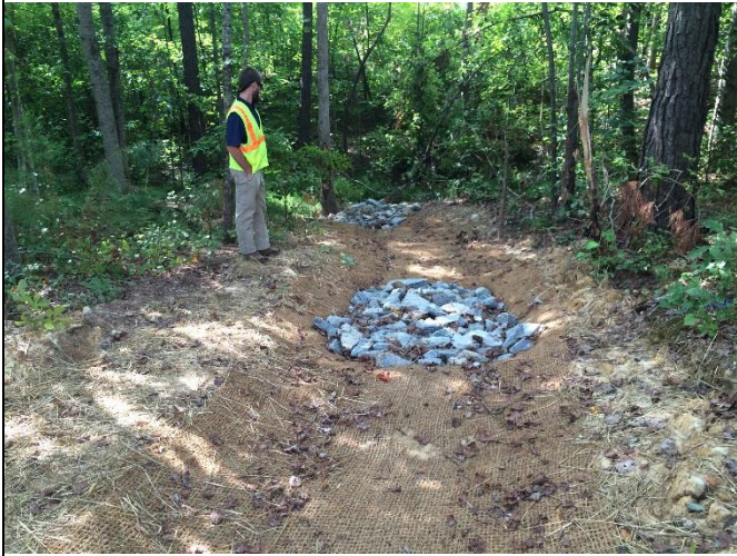
Reach 7, view of stabilized drainage at Station 13+50
