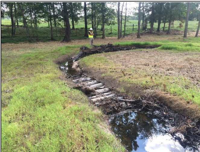
Reach 5, view downstream at Station 31+40
