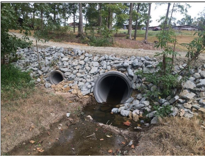
Reach 3, view downstream at pipe crossing, Station 18+50
