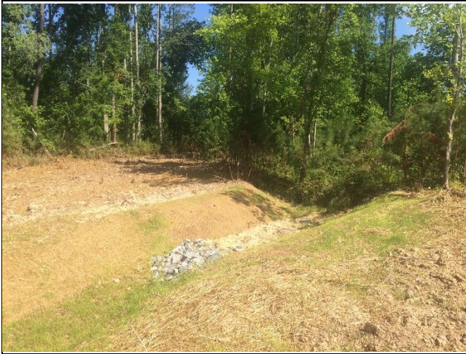
Reach 3, view upstream, Station 11+75
