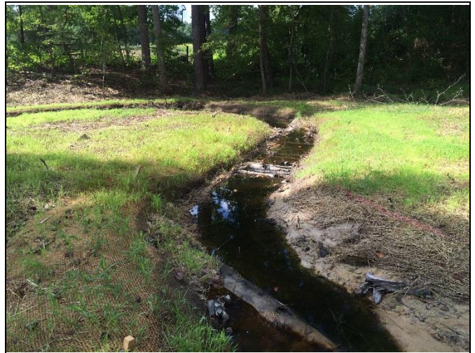
Reach 5, view downstream at Station 30+75
