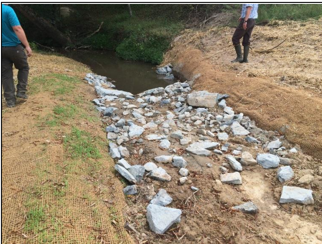
Reach 1, view downstream at Station 43+25
