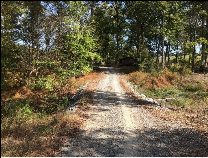
Reach 3, stream crossing, Station 18+80
