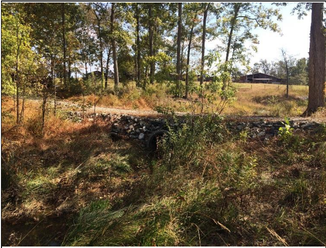
Reach 3, view downstream at pipe crossing, Station 18+50
