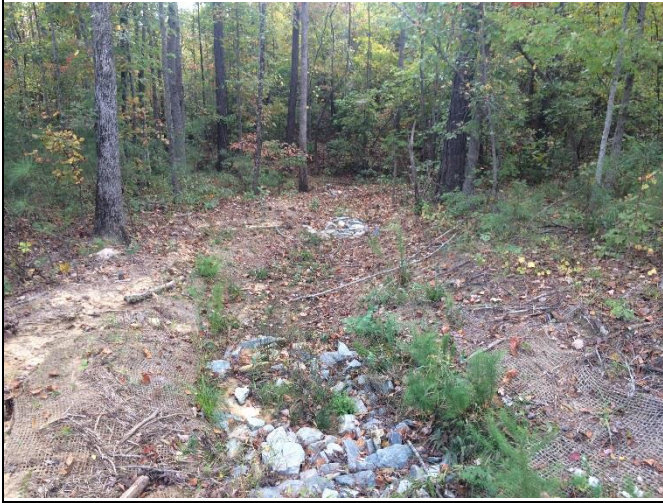
Reach 7, view of stabilized drainage at Station 13+50
