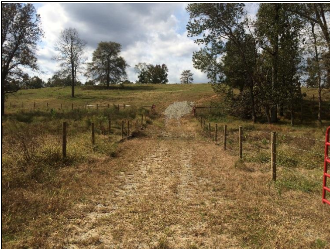
Reach 2, view of crossing at Station 27+75
