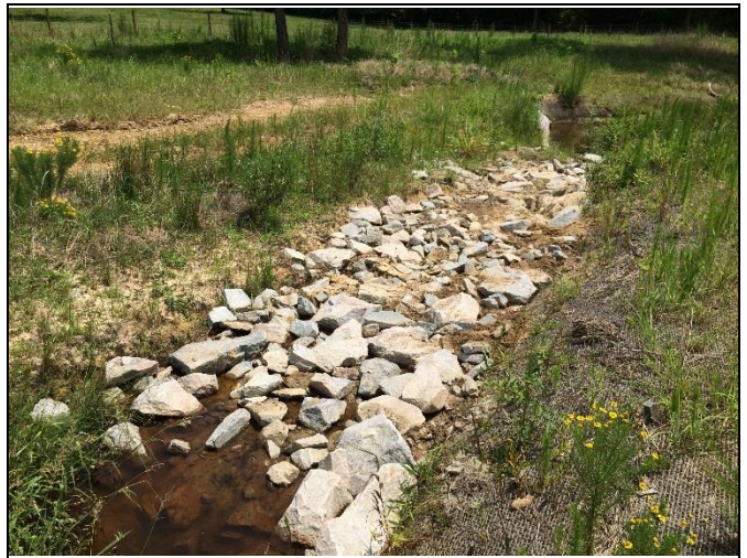
Repaired Stream Area (after), Oct. 2016, Station 42+50
