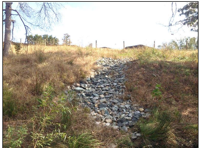
Reach 2, view of stabilized drainage on left bank at Station 20+80
