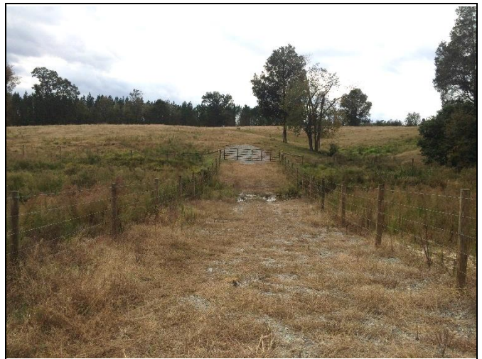
Reach 5, Rock Crossing at Station 35+00
