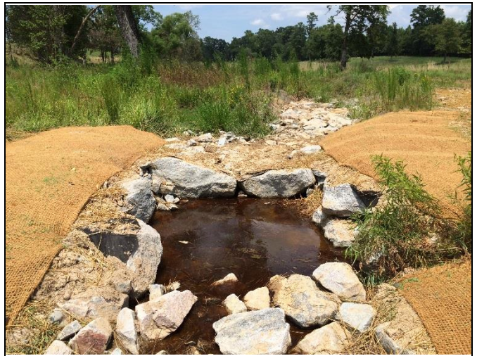
Repaired Stream Area (after), Oct. 2016, Station 42+00
