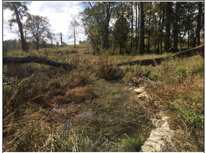
Reach 2, view downstream at Station 25+50
