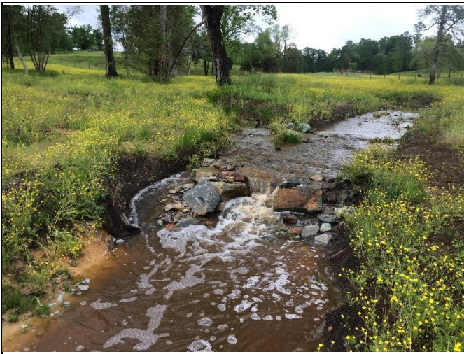
Repaired Stream Area (before), May 2016, Station 42+00
