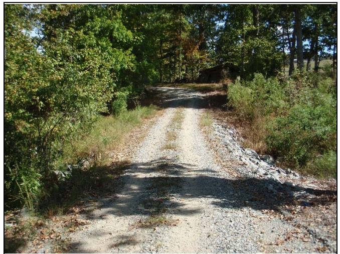
Reach 3, stream crossing, Station 18+80
