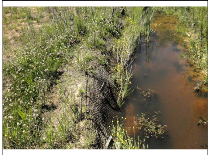
Stream Problem Area 2 (lack of woody vegetation establishment along left bank), R2 Station 34+50
