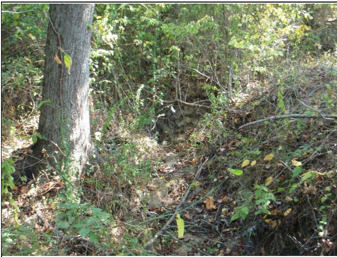
Reach 4, view upstream at Station 10+10
