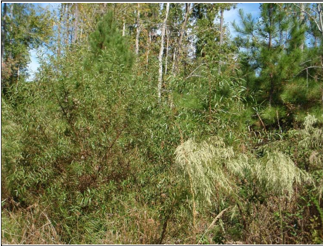
Reach 3, view upstream, Station 11+75
