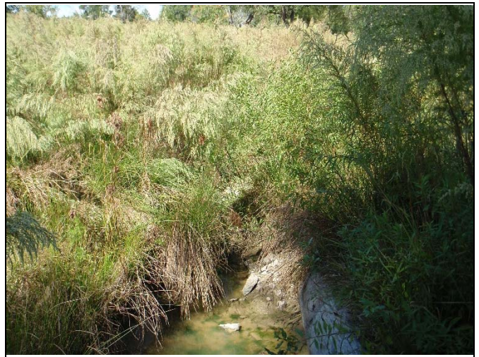
Reach 1, view upstream at Station 42+75
