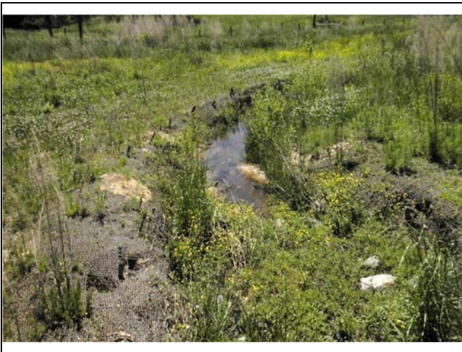
Stream Problem Area 3 (lack of woody vegetation establishment along left bank), R2 Station 35+60
