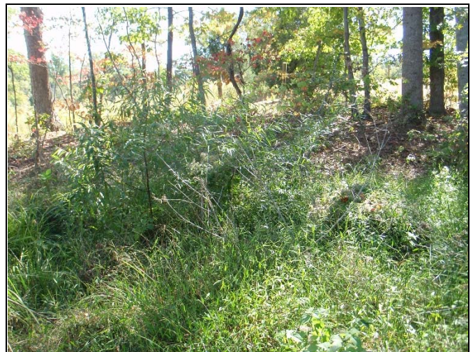
Reach 5, view downstream at Station 32+50
