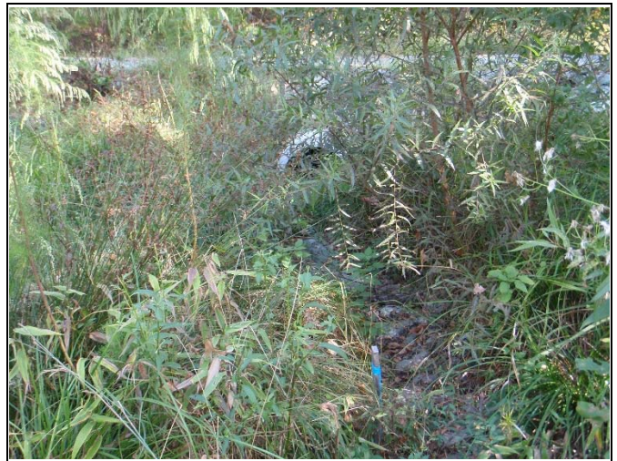
Reach 4, view upstream at Station 10+50
