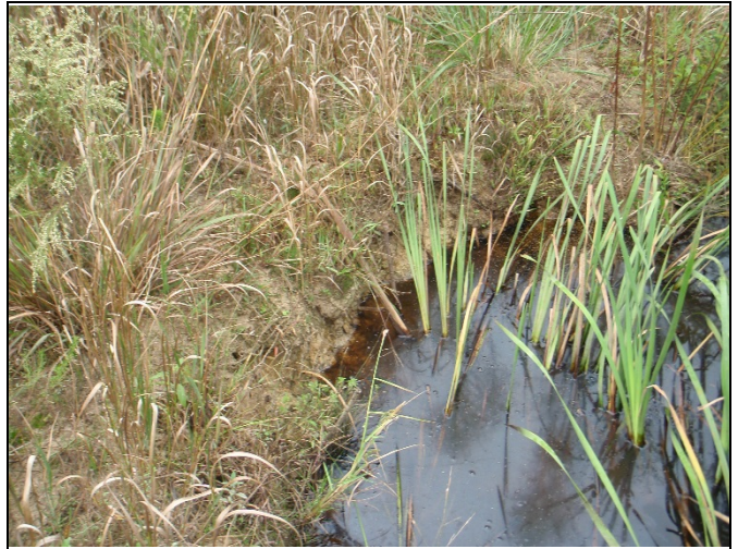
SPA-2: Bank scour and damaged livestock establishment from Hurricane Florence, left bank of R2, Station 35+75
