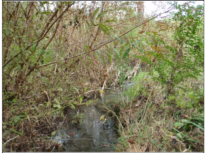
PP-14: Reach 4, view downstream at Station 12+25
