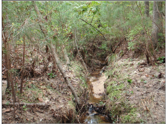
PP-40: Reach 6, view upstream at Station 18+90
