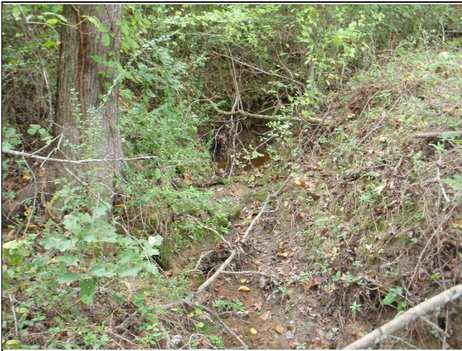
PP-11: Reach 4, view upstream at Station 10+10
