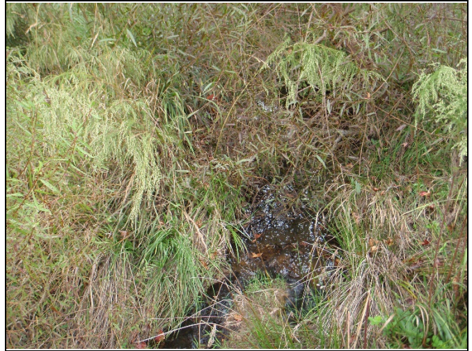
PP-56: Reach 5, view upstream at Station 38+50
