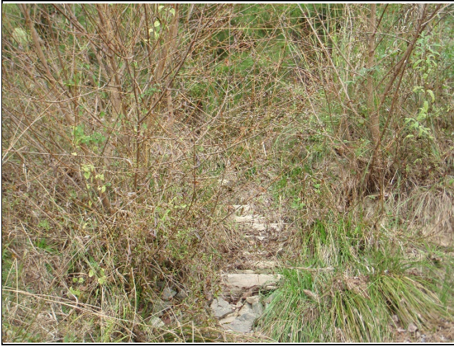
PP-1: Reach 3, view upstream, Station 11+50
