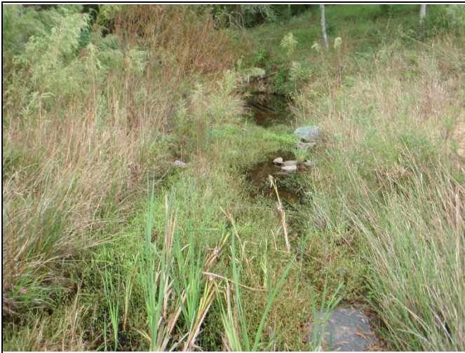
PP-35: Reach 1, view downstream at Station 43+25
