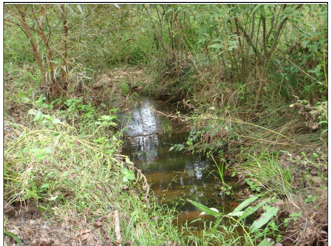
PP-48: Reach 5, view downstream at Station 32+50
