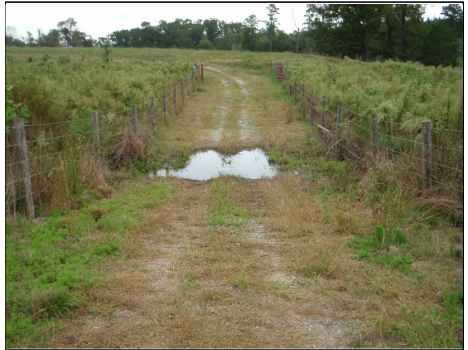
PP-52: Reach 5, view of crossing at Station 35+00
