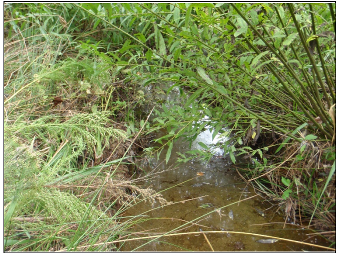
PP-50: Reach 5, view downstream at Station 33+75
