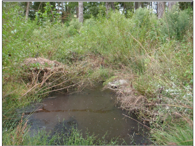
PP-22: Reach 2, view downstream at Station 25+50
