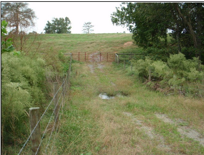
PP-23: Reach 2, view of crossing at Station 27+75
