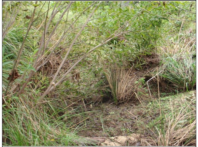
PP-26: Reach 2, view of drainage on left bank at Station 32+90
