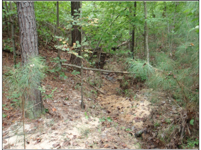
PP-44: Reach 7, view upstream at Station 15+00
