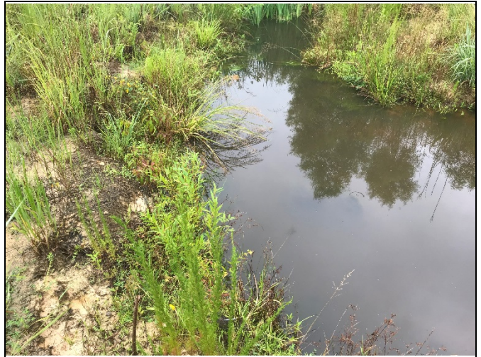
Livestakes planted in March 2018 establishing and stabilizing the left bank of R2, ~Station 34+25
