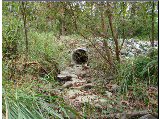
PP-12: Reach 4, view upstream at Station 10+50
