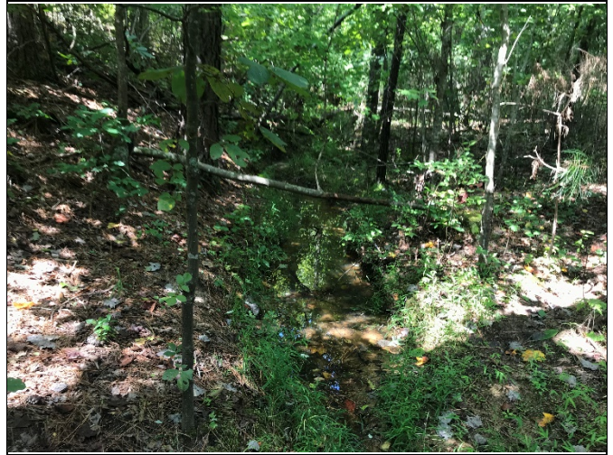
PP-44: Reach 7, view upstream at Station 15+00
