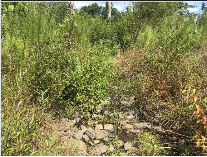
PP-33: Reach 2, view upstream at Station 41+50
