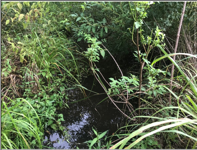
PP-19: Reach 2, view upstream at Station 22+00
