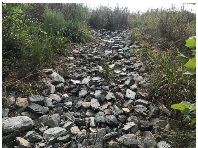
PP-18: Reach 2, view of stabilized drainage on left bank at Station 20+80
