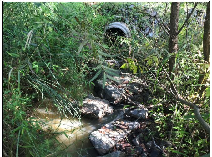
PP-12: Reach 4, view upstream at Station 10+50
