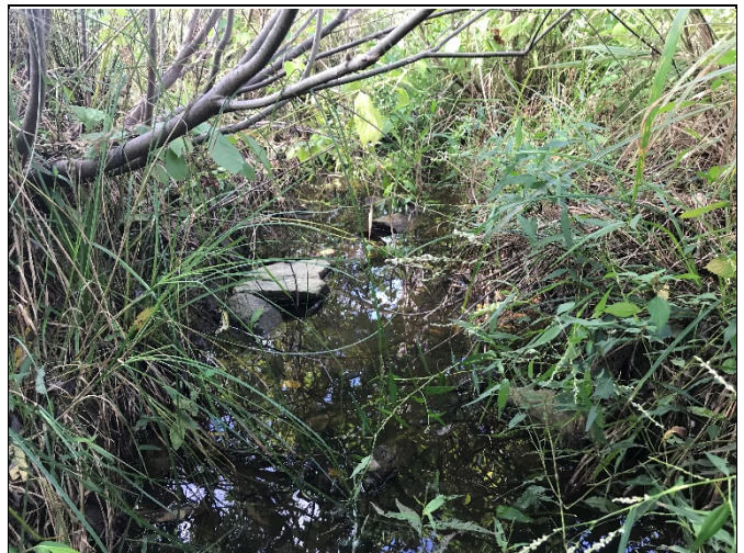
PP-54: Reach 5, view upstream at Station 36+75
