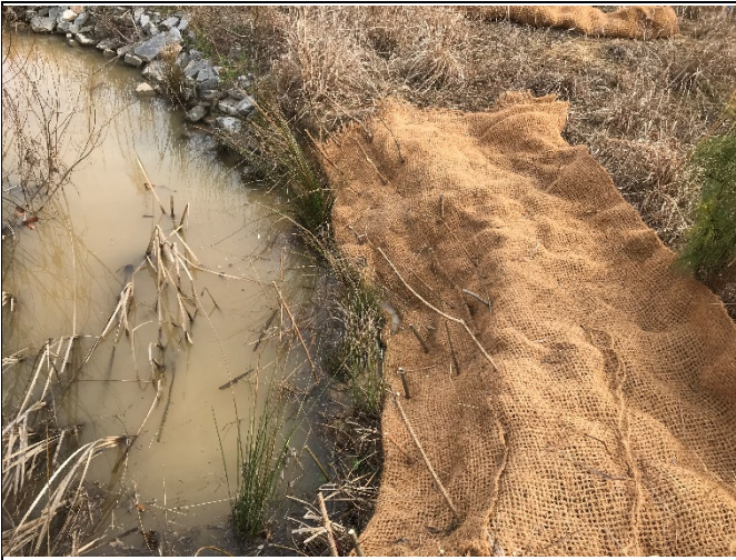
R2 Station 34+75: Bank regraded with matting, seeds, and livestock stakes planted in January 2019 (AFTER)
