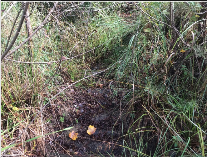
PP-1: Reach 3, view upstream, Station 11+50
