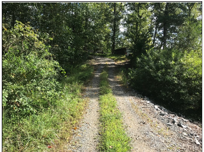
PP-6: Reach 3, stream crossing, Station 18+80
