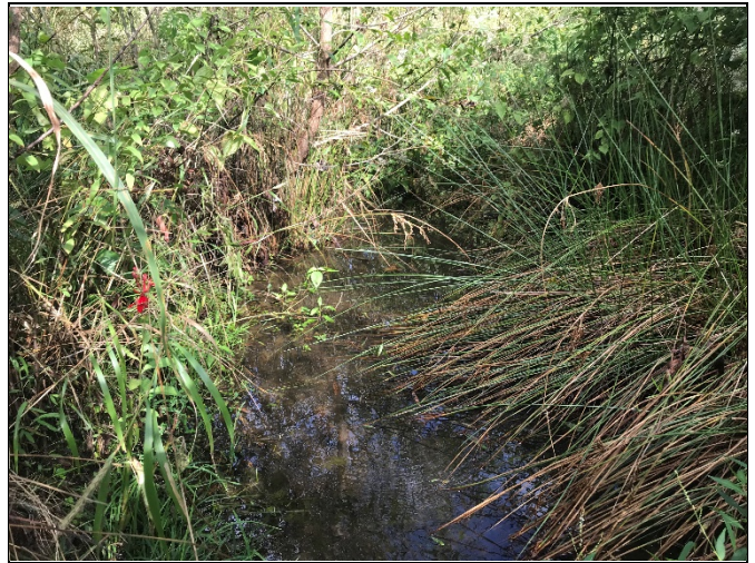
PP-16: Reach 2, view upstream at Station 20+60
