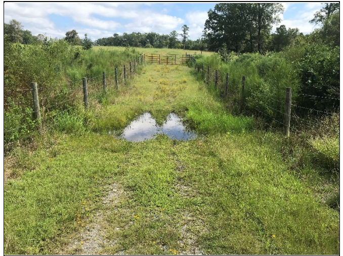
PP-52: Reach 5, view of crossing at Station 35+00
