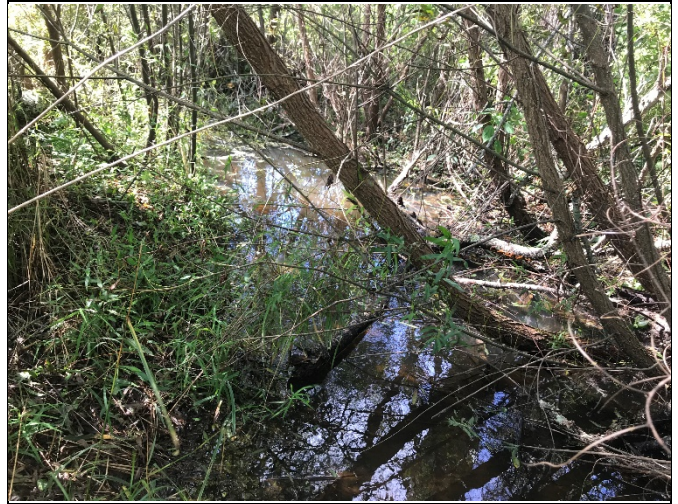
PP-32: Reach 2, view downstream at Station 39+40
