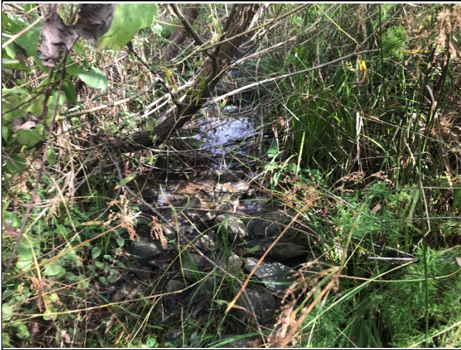
PP-3: Reach 3, view upstream, Station 15+75
