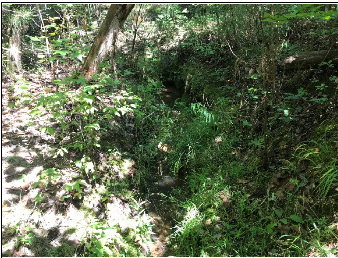
PP-41: Reach 6, view upstream at Station 25+50
