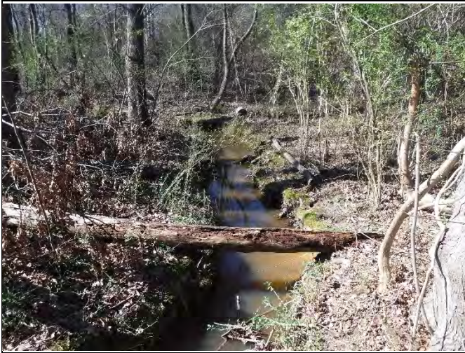
PP-9: Reach 4, view downstream at Station 05+75
