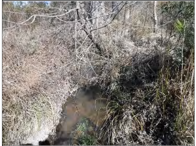
PP-56: Reach 5, view upstream at Station 38+50
