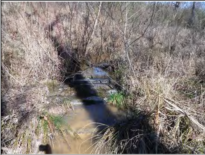
PP-13: Reach 4, view upstream at Station 11+75
