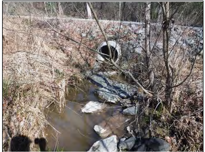
PP-12: Reach 4, view upstream at Station 10+50
