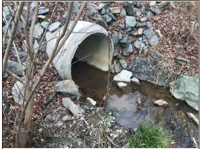
Pipe culvert on R3 (photo: 1/23/20)
