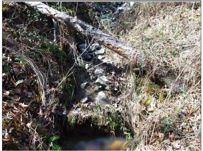
PP-42: Reach 7, view upstream at Station 10+40
