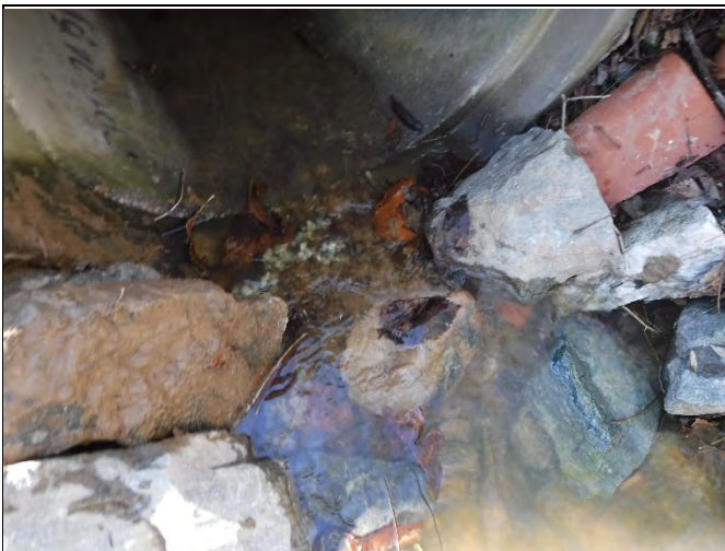
Pipe culvert on R4 (photo: 2/20/20)
