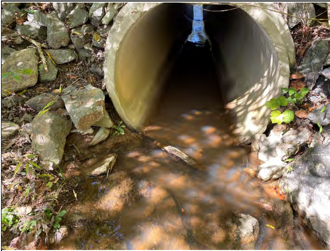
Pipe culvert on R3 (photo: 10/22/20)
