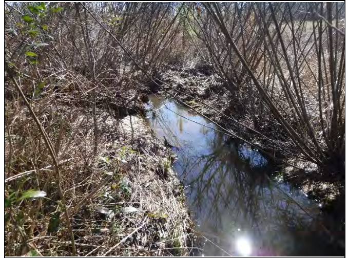
PP-50: Reach 5, view downstream at Station 33+75
