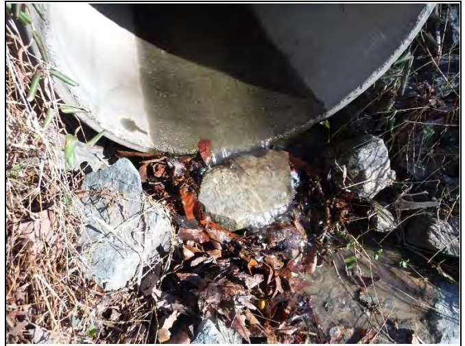
Pipe culvert on R4 (photo: 2/14/20)
