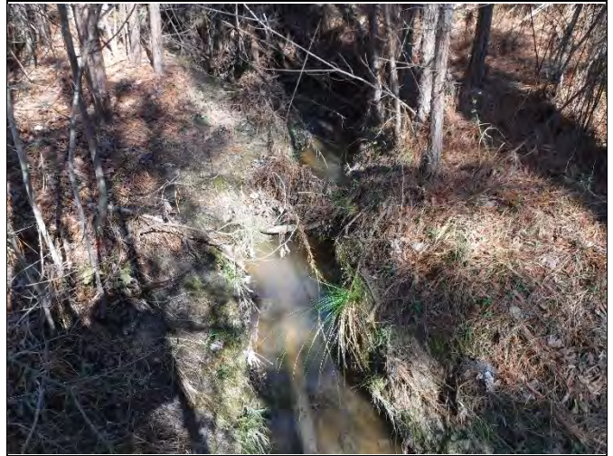
PP-40: Reach 6, view upstream at Station 18+90
