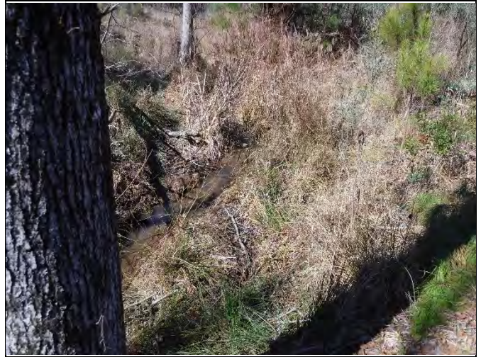
PP-38: Reach 6, view upstream at Station 11+50
