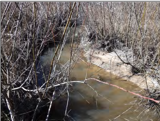
PP-29: Reach 2, view downstream at Station 36+90
