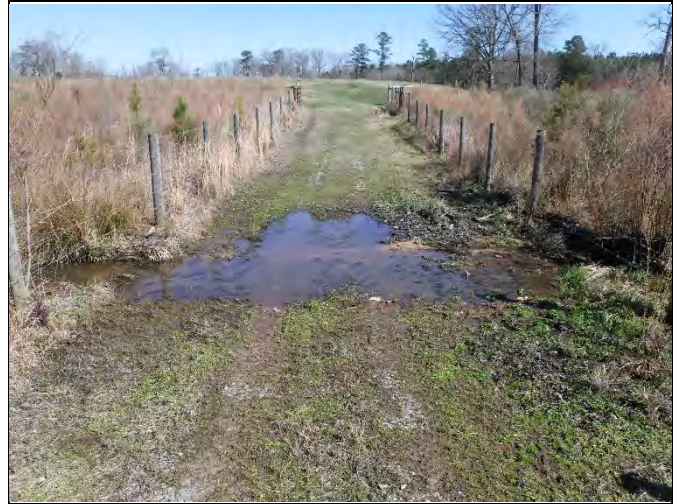
PP-52: Reach 5, view of crossing at Station 35+00
