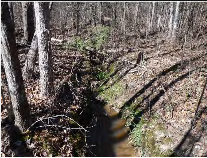
PP-39: Reach 6, view upstream at Station 15+25
