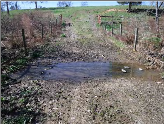
PP-23: Reach 2, view of crossing at Station 27+75
